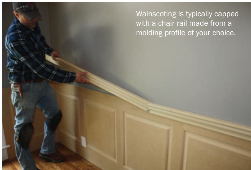
To minimize fastener holes, glue wainscoting panels to the wall and only use enough nails to hold them in place while the glue dries.
