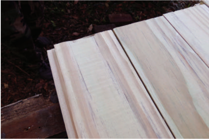
For this repair project we milled interlocking tongue-and-groove boards from treated lumber to replace the original rotted porch boards.
