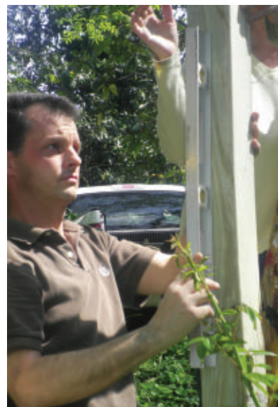
Use a level to check that each post is plumb.
