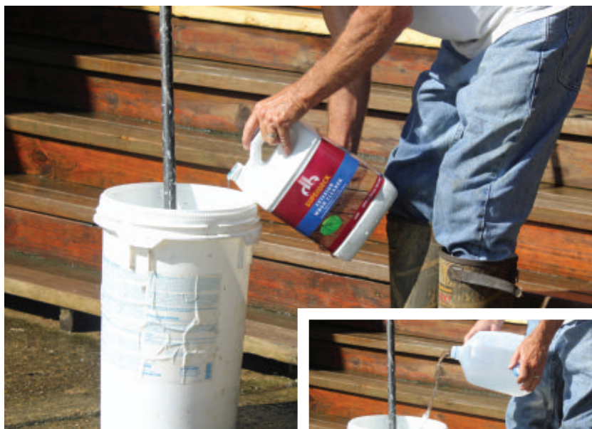
Super Deck Exterior Cleaner concentrate is used to clean the wet areas.
