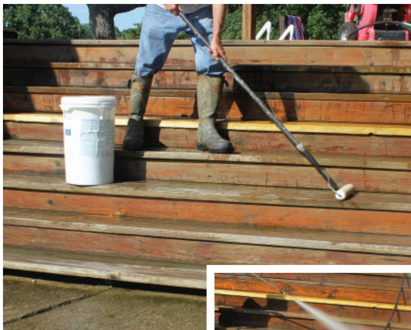
The diluted cleaner is applied with a roller.
