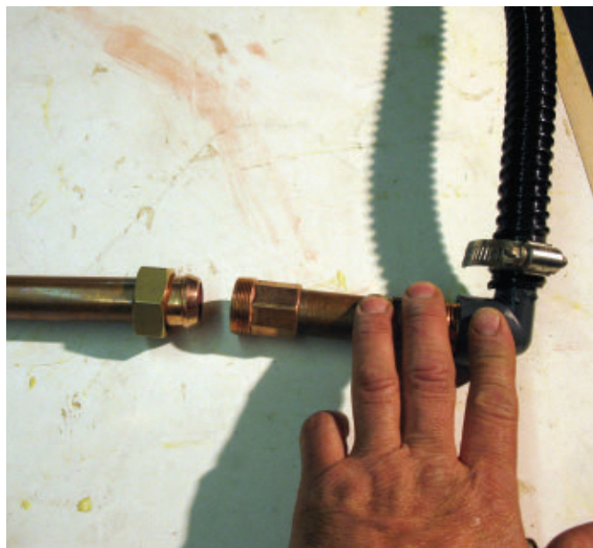
A short piece of 3/4" pipe separates the male adapter from my disconnect fitting. The disconnect fitting will allow me to drain the pot and remove it for winter storage.
