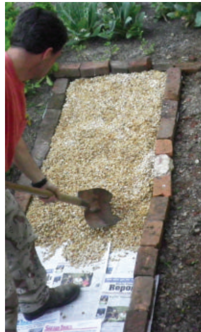
Hand-shovel pea gravel into the paver-lined walkway to keep from spilling it into the growing areas of the garden.
