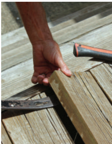
Old boards, or sections of boards, are then carefully pried out.
