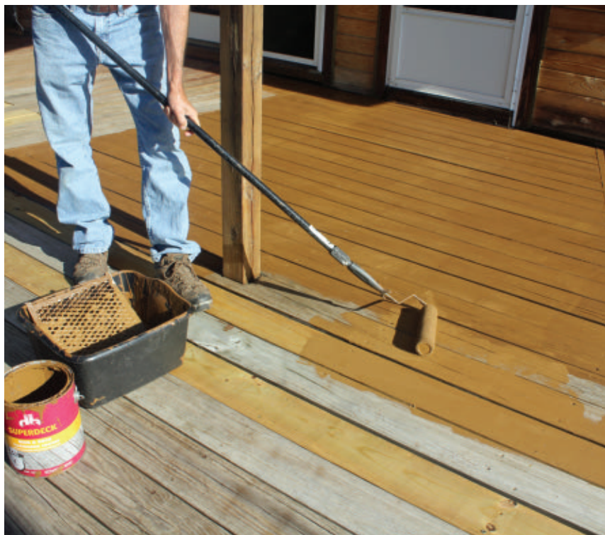
For the last coat Duckback Anti-Skid additive is added.
