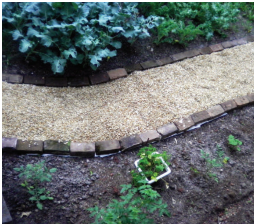
The finished walkway provides access to plants while preventing compaction of the soil in the growing areas. Simple brick pavers are used to retain the pea gravel.
