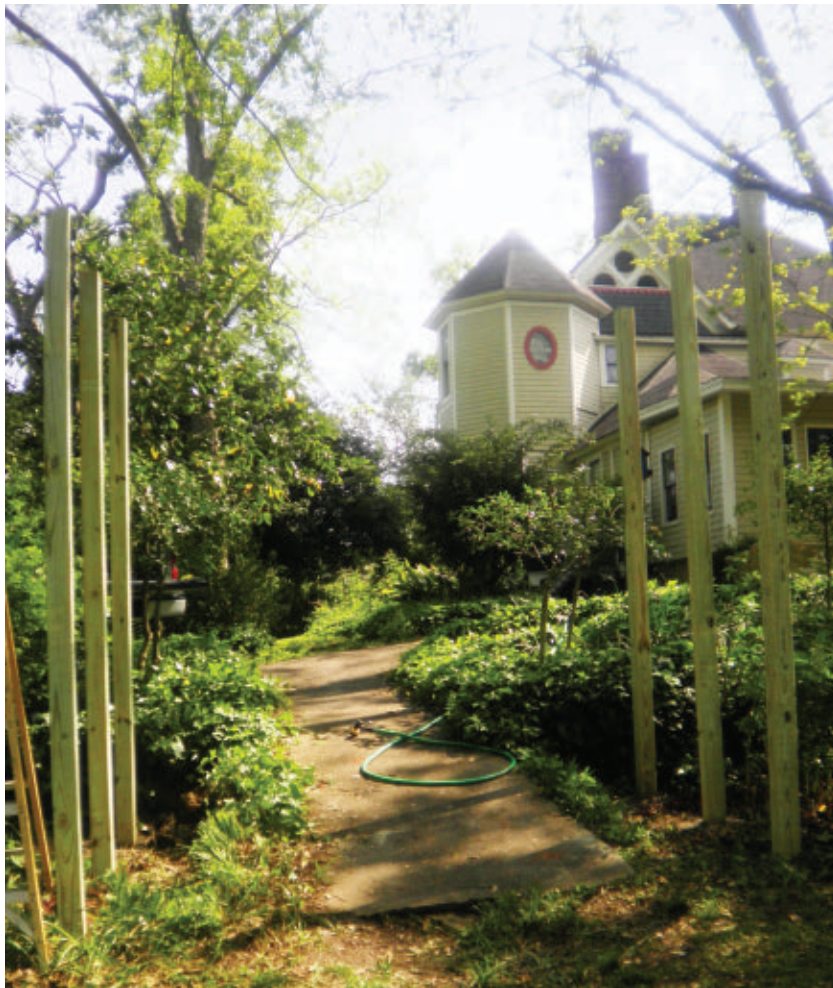
The arbor is supported by two rows of three equidistant 4x4 posts.
