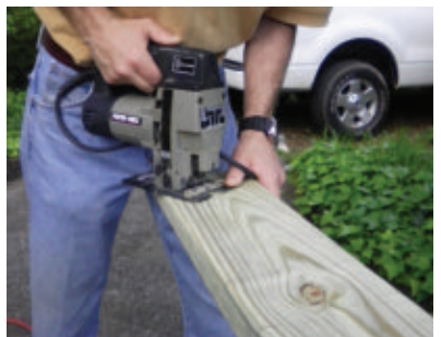
Cut the curved profile with a jigsaw.
