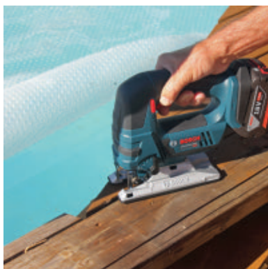
Old pool-surround edging screws were too rusty to remove, and had to be cut out using a saber saw and metal cutting blade.
