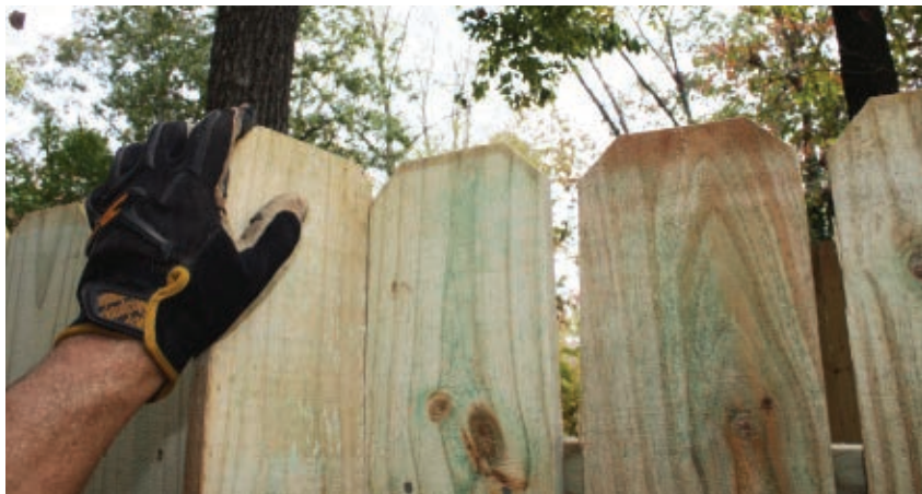
We used the edge of a fence board as a spacing block.
