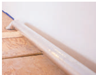
All joints are sealed with aluminum tape.
