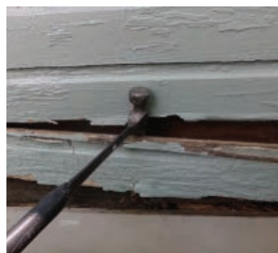
We pried off the rotted siding and used its profile as a template to mill the replacement pieces.
