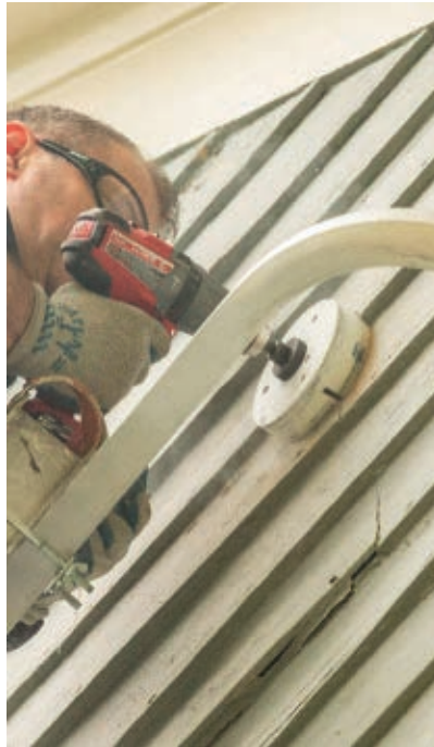
Use a hole saw to cut passage for the duct.
