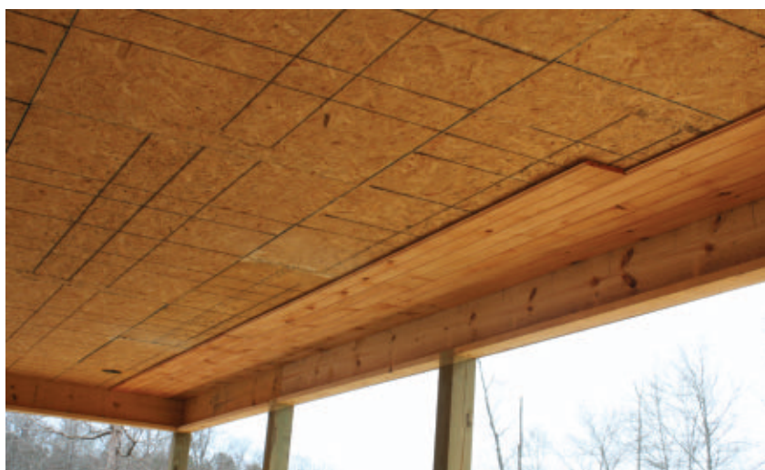
Begin in one corner of the starting row and stagger the end joints between rows.
