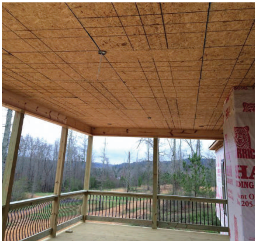
Lively installed a 1/2" plywood sub-ceiling over joists on 12" centers.
