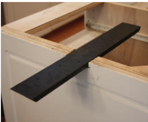
Granite countertops that have an overhang will need a countertop support to carry its weight from below.
