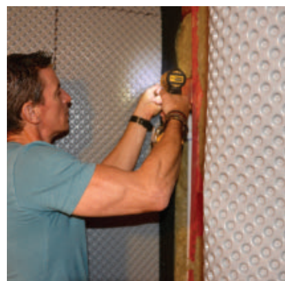
A layer of Dam Proofing Membrane (DPM) covers the roofing membrane and framing.
