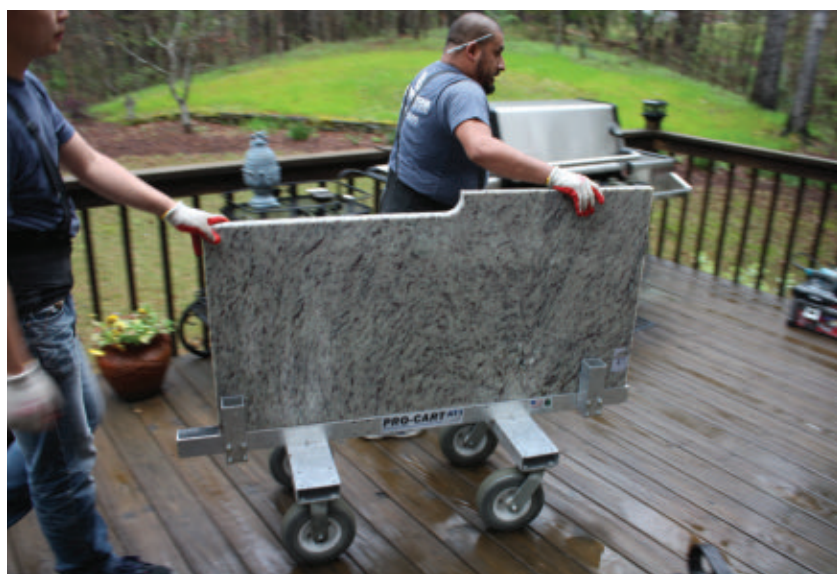
Once on location, the installers use wheeled carts to move the heavy slabs around the site.
