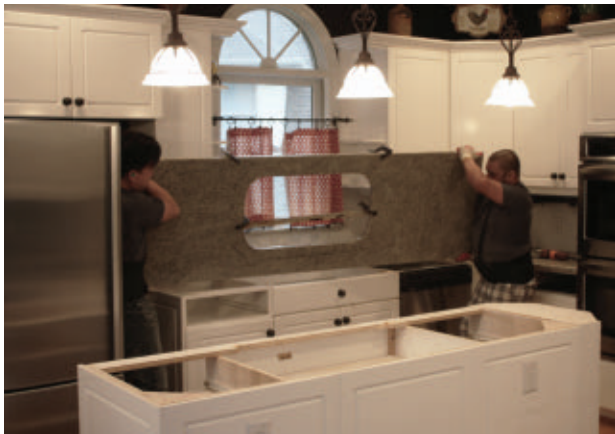
This L-shaped counter required two sections seamed together.
