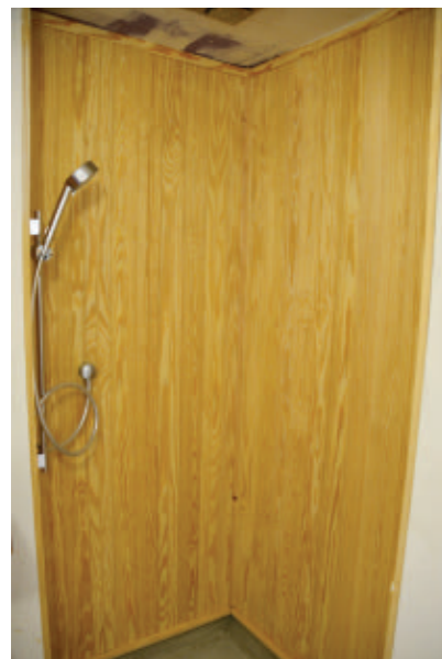
Shown here is the completed cladding.
