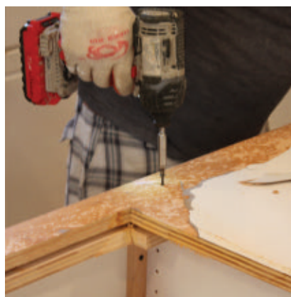
Pry up the old laminate and remove any screws hidden beneath it.
