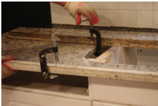
Note the angle-iron bracing clamped across the length of the countertop to stabilize and reinforce its shape. This is particularly important for the section with the sink cut-out, which has a weakened center area since the granite is missing.
