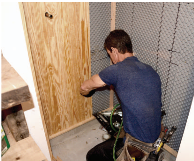
After coating their backs with Spar urethane, the tongue-and-groove cladding is installed as the shower surround.
