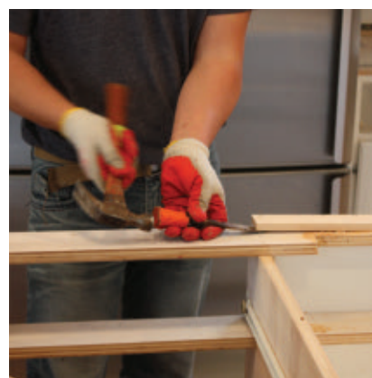
Pry off any old wood blocks or shims from the top of the cabinet base.
