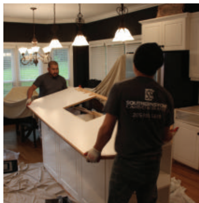
With all screws removed, the countertop should lift freely off the base.
