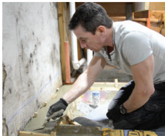
The wood shower began with the concrete curb poured into a form on the basement slab.
