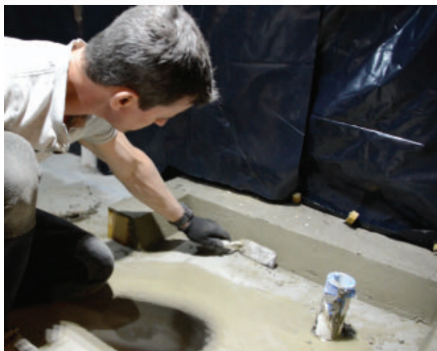
The curb directs all the shower water away from basement walls and toward the drain.
