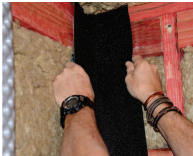
After the shower area is framed with wood studs and insulated, roofing membrane is installed at the corners.
