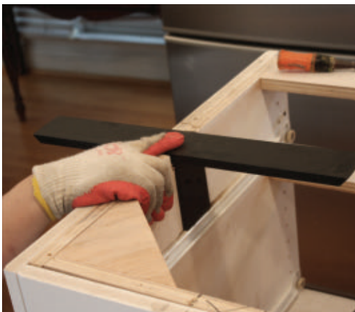
This support extends inside and outside the kitchen island's cabinet base
