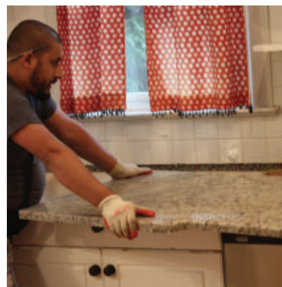
Carefully set the new granite countertop section in place on the cabinet base.
