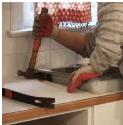
First step in removing an old countertop is to disconnect all integrated appliances.
