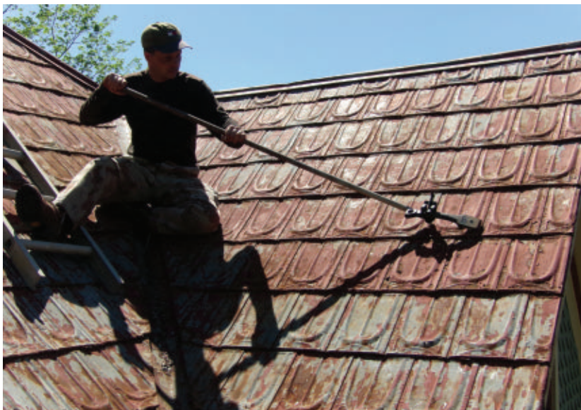
This terne metal roof had hips and valleys that complicated the project.
