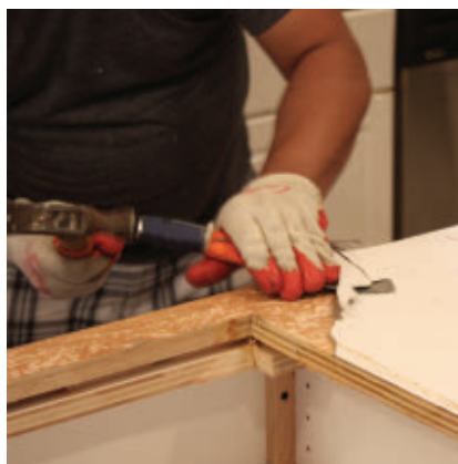
In some cases, a countertop may have been fastened to the cabinet base prior to having the finished surface installed.
