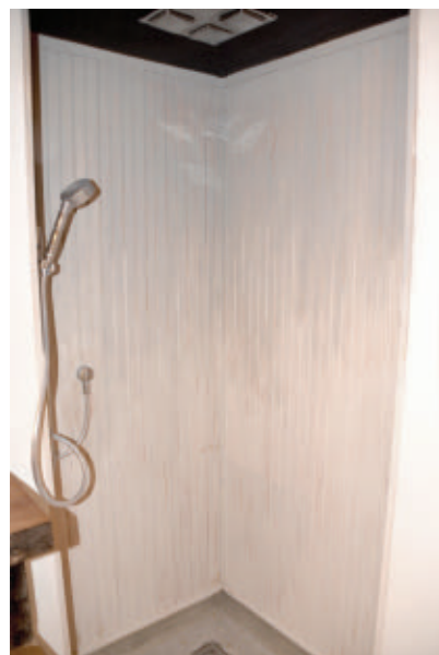
You have a number of water-resistant finish options for the shower panels. The finish shown is called an ombre effect, which lets the natural feel of the wood ripple through the color.
