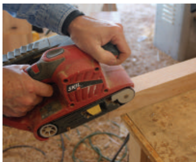
Any irregularities in the leg cuts are sanded smooth.
