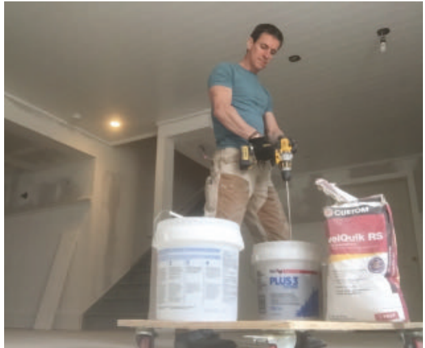
If you have dips in the subfloor deeper than 1/4", mix up some floor leveler and apply it as needed.
