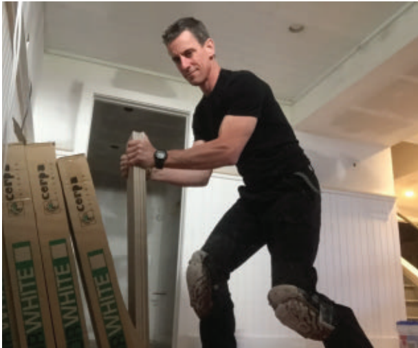
For this job, we installed TileBar's succulent wood-themed large format Cerpa Arena plank tile.
