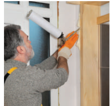
Expanding foam is a popular sealant for unfinished areas of the home that will be covered with trim.
