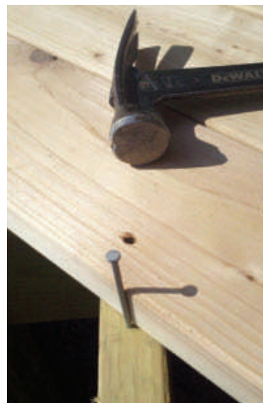
Kiln-dried lumber like Western Red Cedar should be gapped during installation to give room for expansion and contraction.
