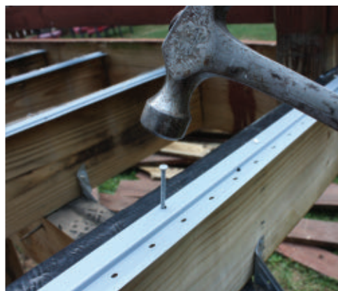
Nail to the tops of the joists.
