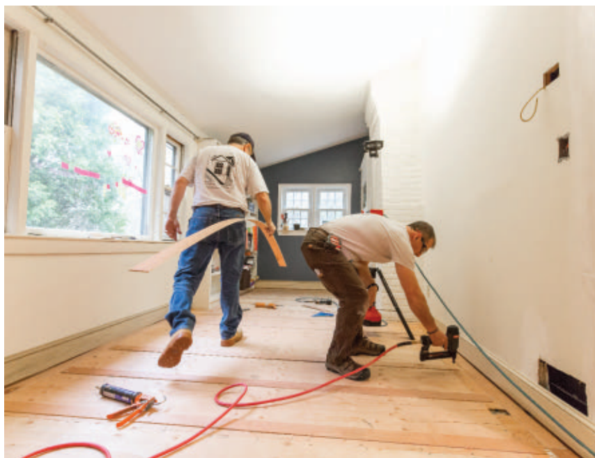
The sleepers were spaced 16" on-center, which creates a 10" wide space between them to run three loops of radiant cable spaced 3" apart.
