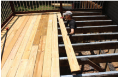
Stagger the end-joints from row to row.
