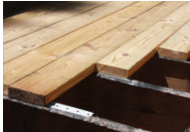
Inspect the end-grain of the boards and fasten them “bark side up.”
