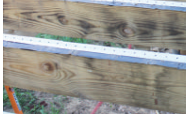
Nail to the tops of the joists.
