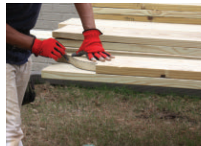
After deciding on a rafter-tail pattern, cut the first rafter and use as a template to mark the others.
