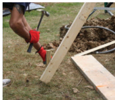
Stake the the post braces to the ground to hold the posts in place while the concrete dries.
