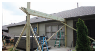
Use 2x4 braces to hold the support structure plumb and square while building the pergola.
