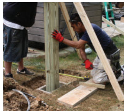
Setting the posts square and plumb is a two-man job.
