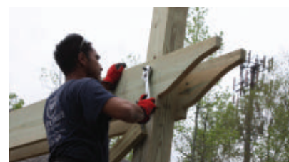
Fasten each corner assembly with two 1/2" lag bolts, washers and nuts.
