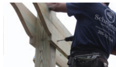
Make the final connection by drilling two 1/2" pilot holes through the posts and double girders.
