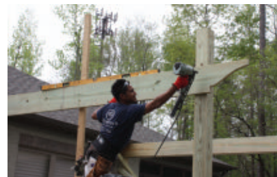
Install the girders level across the side posts.
