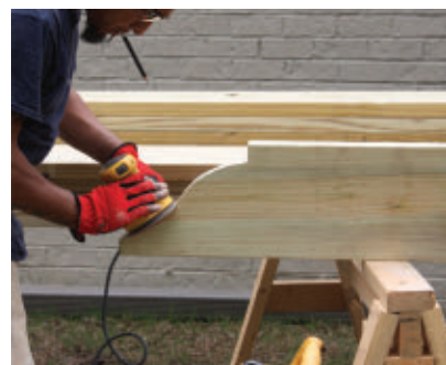
Sand the profile to prevent splintering.
