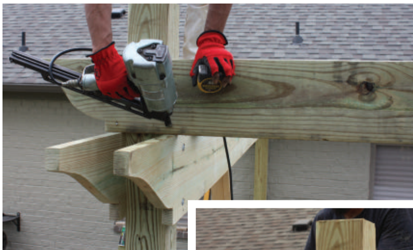
The rafters bridge over the girders at 90 degrees.
