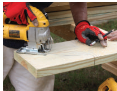
The thin blade of a jigsaw cuts the curved profile.
