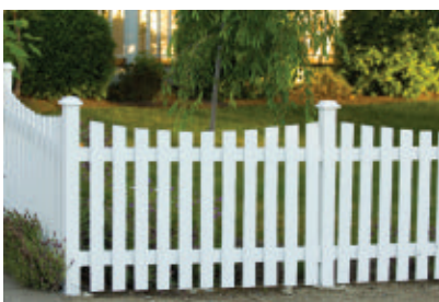
Capped fence posts and a gentle curve cut in the top of the pickets give this fence its character.
