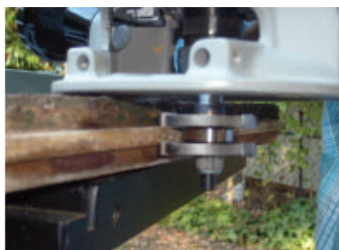
Use an old board as a template for the tongue-and-groove joints, and rout the new joints along each replacement piece.
