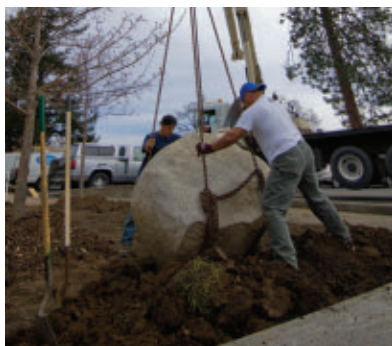
After digging a hole with a backhoe, the crew directs the crane operator to set the rock in the hole.
