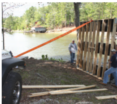
We used a Jeep equipped with a winch to help flip over the 10x10' foot platform. The winch was critical to manage the heavy weight of the structure.
