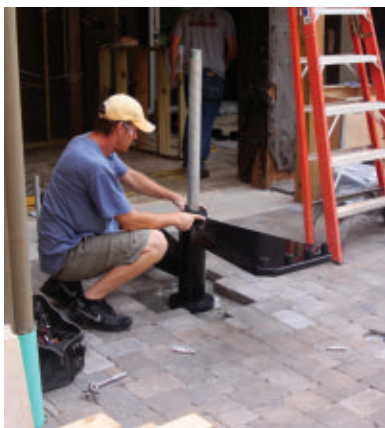
The treads and spacers slide over the pole.
