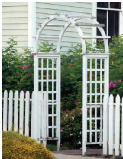
Gate openings can be handled in a variety of ways. A cleaner approach here could have incorporated the fence posts on each side of the arched trellis into the trellis design.
