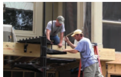
The next step is baluster installation.
