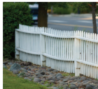
You know not to lay fence rails flat, right? The structural strength is lost resulting in sagging fence rails and sinking pickets. At least the builder was consistent so the resulting sag creates its own pattern.
