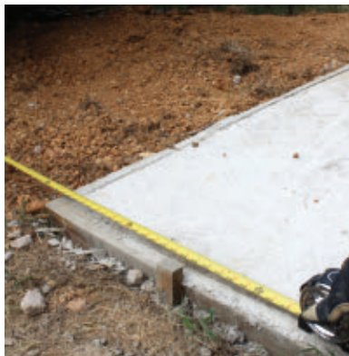
Measure the run from the plumb mark to the landing.
