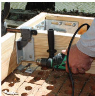
The dock joists install with heavy-duty plates and through-bolts. It helps to clamp the hardware in place while you drill the bolt holes.
