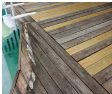
The rebuilt deck with old and new boards. Note the rot on the pool edges, these boards haven't been replaced yet.
