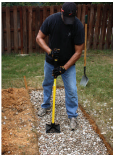
My first step was to excavate the slab location and tamp down a bed of gravel for the concrete.
