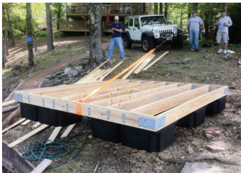
We used a Jeep equipped with a winch to help flip over the 10x10' foot platform. The winch was critical to manage the heavy weight of the structure.
