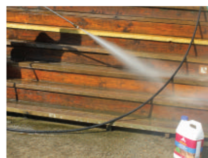
The deck is brush-scrubbed and power-washed.
