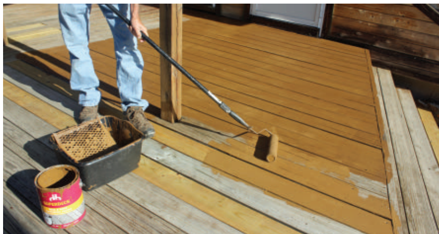
The Superdeck Deck & Dock is rolled onto the cleaned, dry surfaces.
