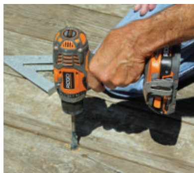
Starting holes are bored in the corners of the mark.
