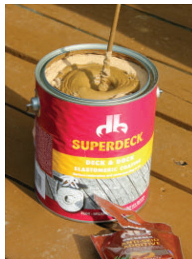
The additive must be thoroughly mixed into the coating.
