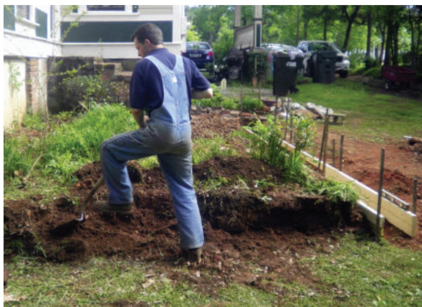
The wall was reconstructed from a round shape into two straight walls that intersected at right angles.
