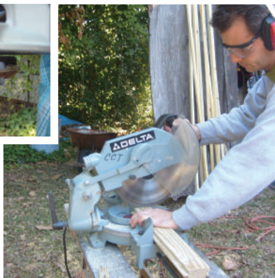
Cut the replacement boards to length.
