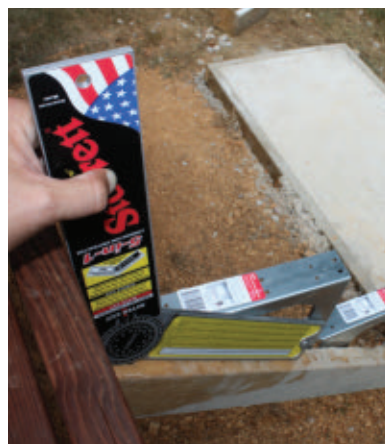
I tacked up a temporary 2x4 stringer to help check all my measurements.
