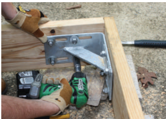
We began construction on the relatively flat driveway to keep the rim-joist frame as square and level as possible.
