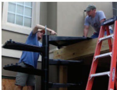
The staircase shown has a mezzanine landing.
