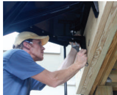
Attach the landing to the finished floor with the included hardware.
