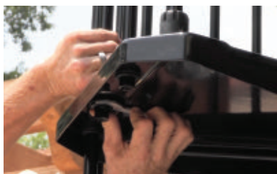
Once in position, the balusters can be secured from beneath the treads.
