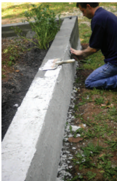
The wall was coated with surface-bonding cement to make it stronger and provide a finished texture to the outside of the block wall.
