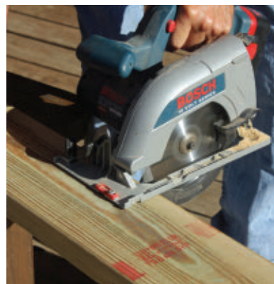
A cordless circular saw makes quick work of cutting deck boards to length.
