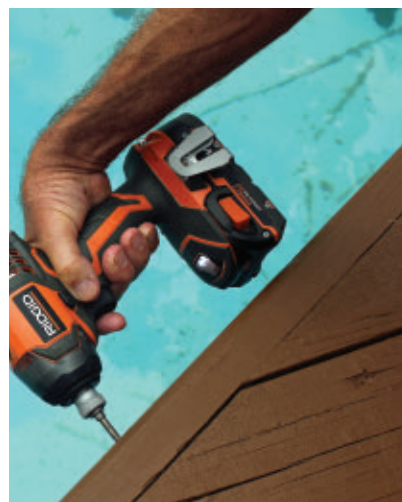
Pool edging has routed rounded edges, and 15-deg. angles are cut using a miter saw. The trim is installed with screws.
