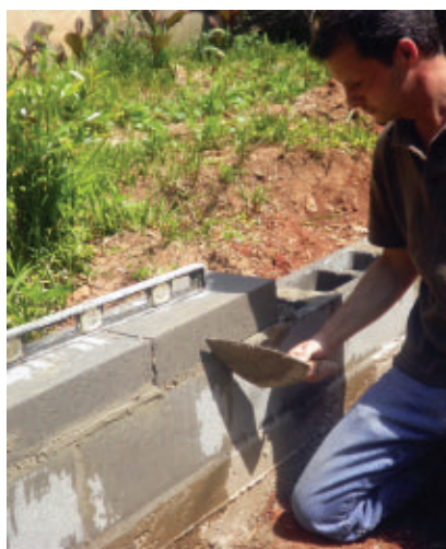
The 4" thick cap blocks provide a finished look to the wall's top course.
