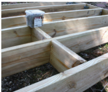
We installed 2x8 blocking between the three center joists that would not be bridged by the floats.
