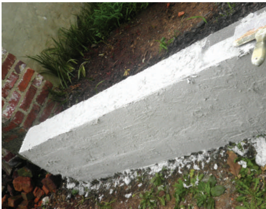
Apply the surface cement with the blade held almost flat against the surface of the wall to achieve a stucco-like finish.
