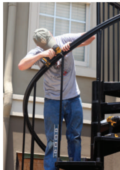
The handrail installs with the same corresponding curve of the staircase.
