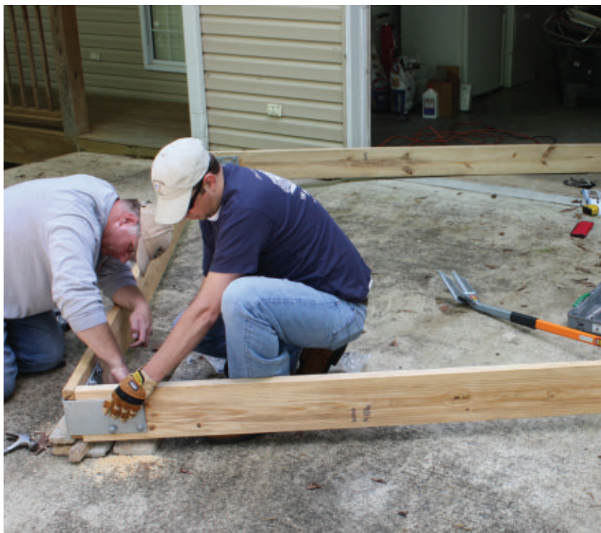
We began construction on the relatively flat driveway to keep the rim-joist frame as square and level as possible.
