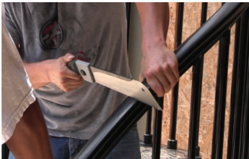
The handrail can be trimmed to fit.
