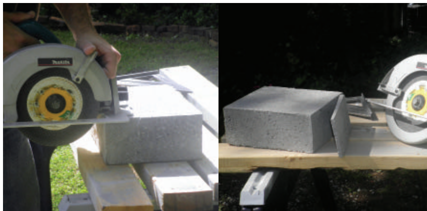
A wet saw does the best job of cutting concrete and block, but occasional cuts can be made with a handheld circ saw equipped with a carbide blade.
