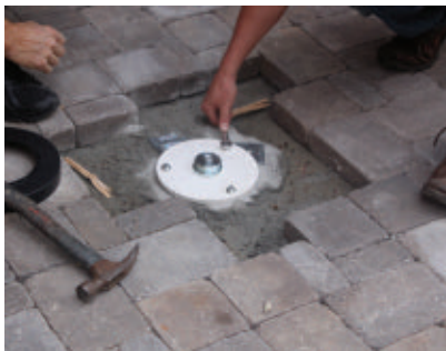
Install the base plate.
