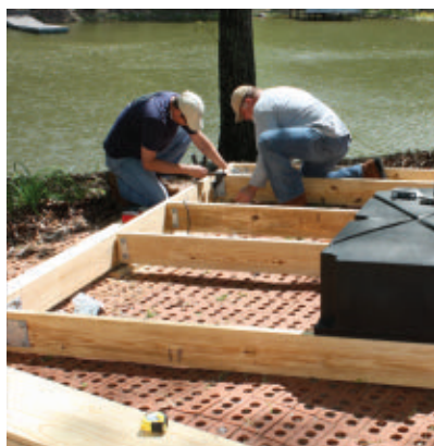
After locating the joists on which the flotation devices will mount, we spaced the remaining joists 16" on center.
