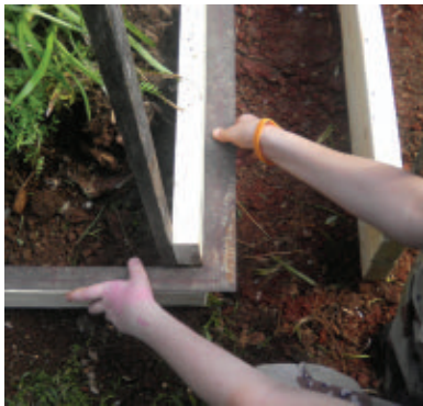
A framing square helps to ensure the angle is true when building the concrete forms.
