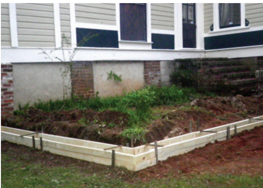
Shown here are the completed forms, made from 2x lumber, staked securely to the ground and bridged with oak ties.
