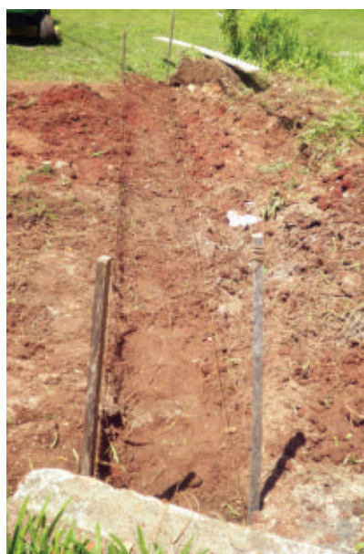
First, dig the trench for the wall's concrete footing form.
