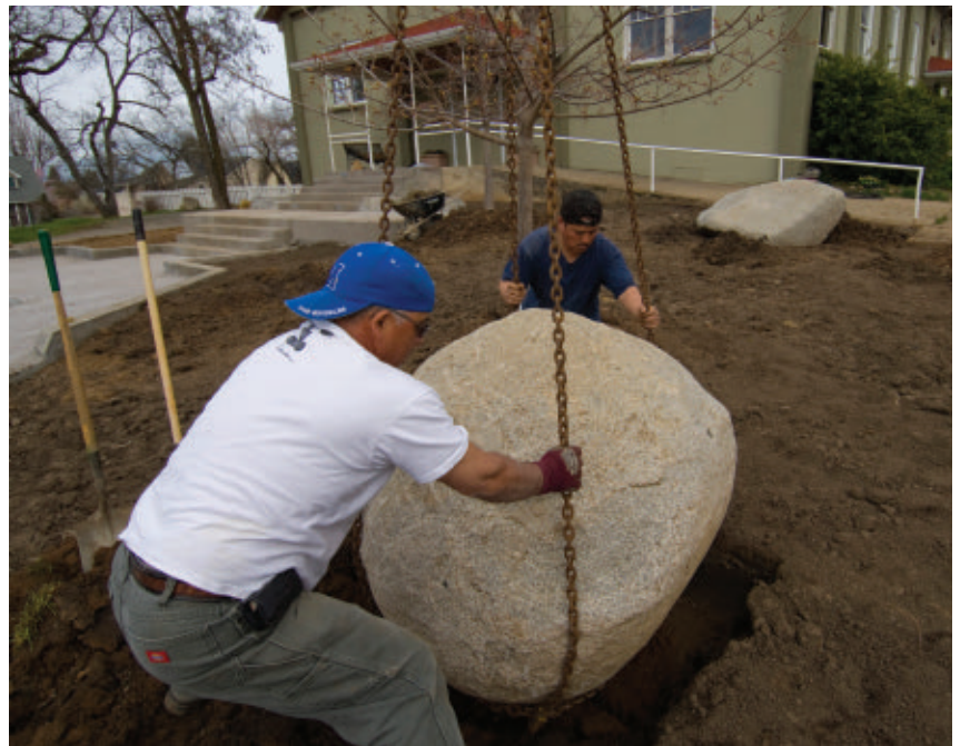
One of the advantages of this rigging setup is that the rock can be easily turned to position it in the desired direction.
