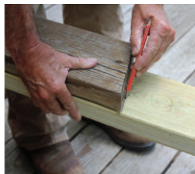
The removed boards with angled cuts are laid on new boards to mark the cuts.
