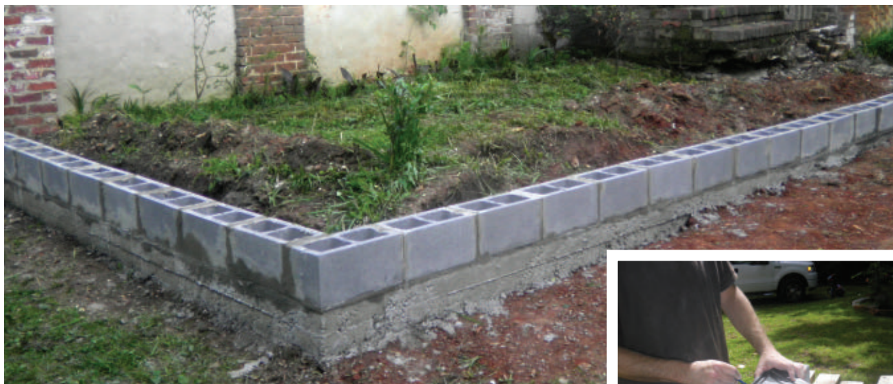
The wall consisted of the concrete foundation, a full course of cement block and an upper course of solid cap blocks.
