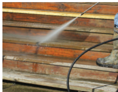
The deck and steps are lightly power-washed.
