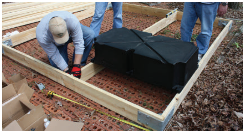
Make sure to locate the joists so they match the mounting holes of the flotation devices.
