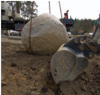
Leaving a large round rock sitting on the surface was not the look Ashland wanted, so his crew used an excavator to dig a hole for the bottom half of the rock.
