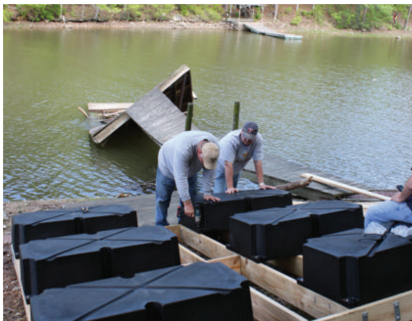
A total of six 2x4' floats were required for the swimming dock. Notice the old storm-wrecked dock in the background, which provided the motivation for this project.
