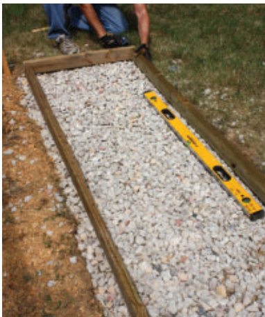
The concrete form was made from 2x4s.
