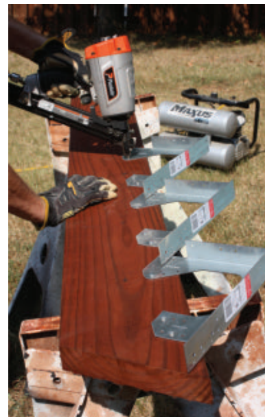
I tacked the stair brackets in place with nails before securing them with screws.
