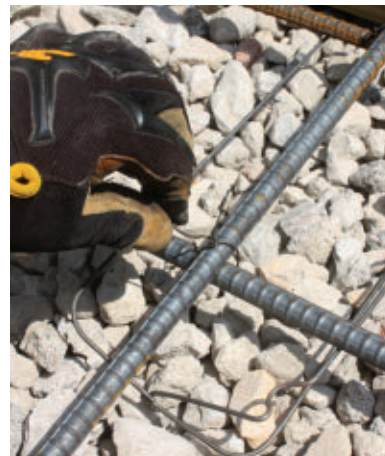
Secure the rebar grid with wire ties.
