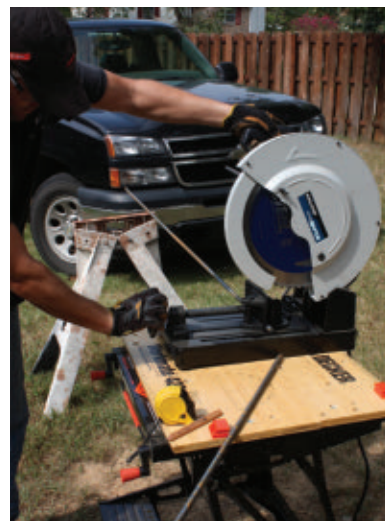
I used a cutoff saw to trim the rebar to size for the reinforcement grid.
