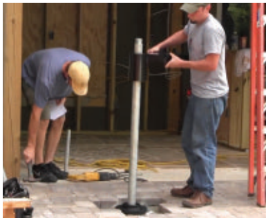
Fasten on the base-plate cover and screw on the center pole.
