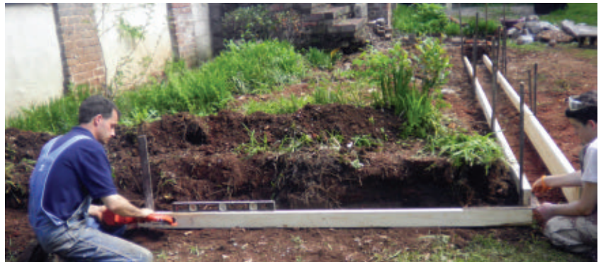
Check and recheck the forms for level and plumb. A perfectly flat foundation will determine the layout for everything that is placed on top.
