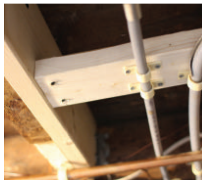
Extra blocking was added between joists to support overhead pipes.
