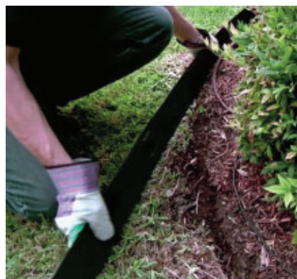
Place the edging in the trench.
