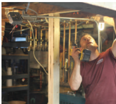
Use an impact driver to screw them in a staggered pattern throughout its length.
