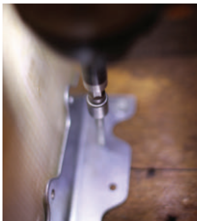
Fill all holes in the hanger with screws.
