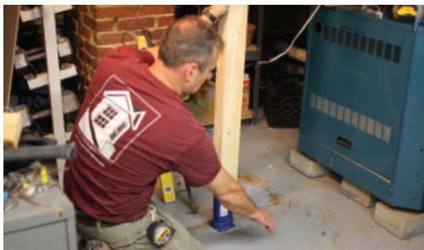
Slowly raise the jack. A good rule of thumb for floor joists is to lift them no more than 1/8" per day.
