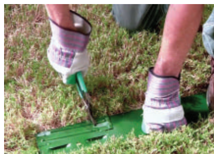
Pry off the stakes with Channellock pliers.
