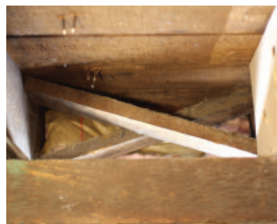
The length of the new joist was cut so the end fit 3" over the support beam.
