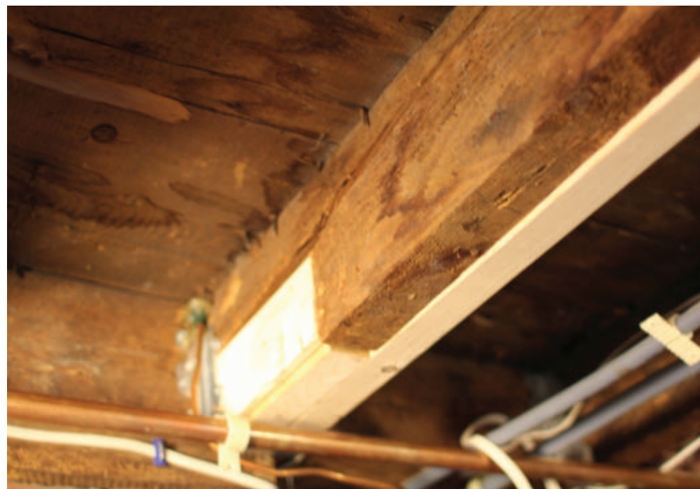
Use an impact driver to screw them in a staggered pattern throughout its length.
