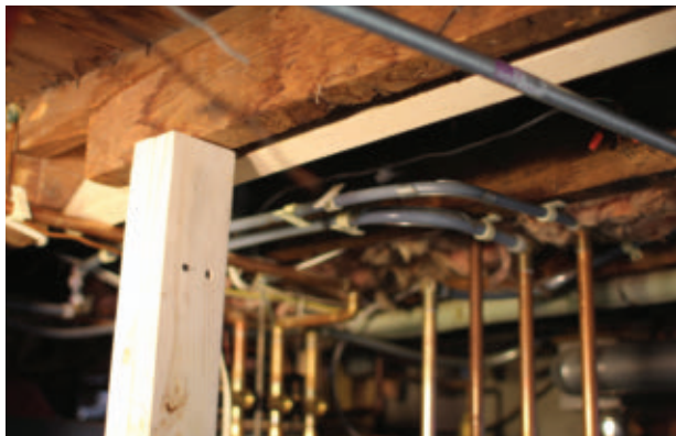
The jack post is simply two 2x4s nailed together.
