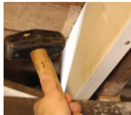
Level the joist before fastening.
