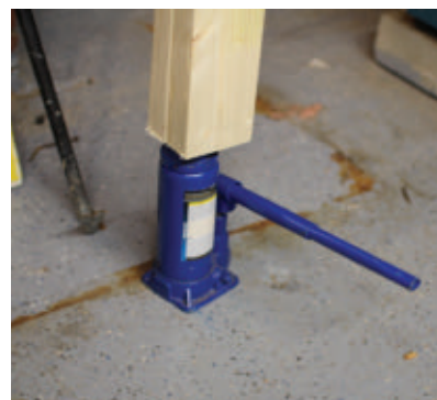
You can raise the existing joist with a bottle jack and jack post.
