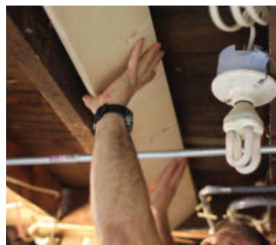
"Sistering" the joists means to fasten the joists together through the face to double the thickness of the framing.
