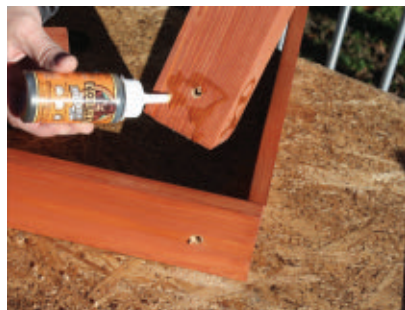
Apply high-quality polyurethane glue to all mating faces.
