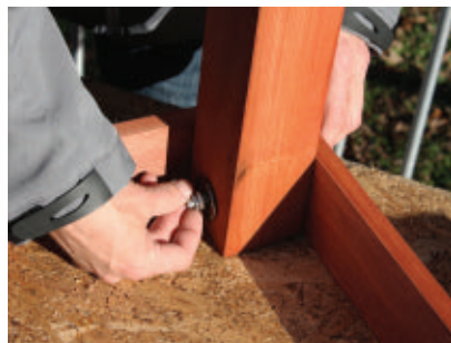
Insert the carriage bolt through the front/side boards and the legs, and then tighten with a nut and washer.
