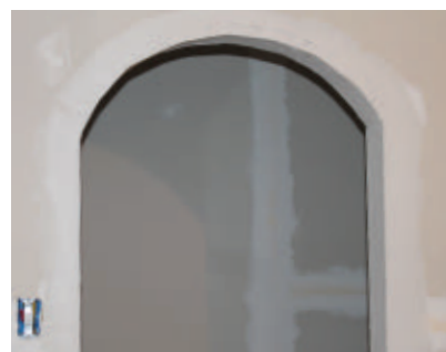
The doorway was then finished with joint compound, primed and painted.
