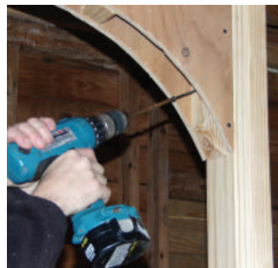
Fasten the archway to the framing with 3" drywall screws.
