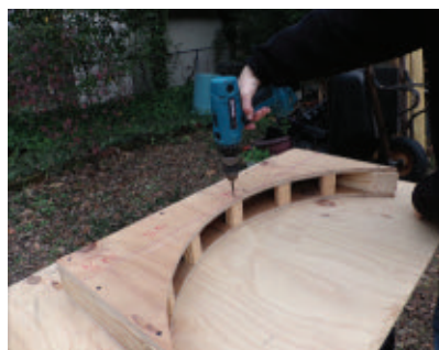
Screw the blocking in place but leave out the end pieces until the archway has been installed.
