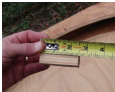
The blocking will have to be trimmed from 2x4 lumber to fit between the panels.
