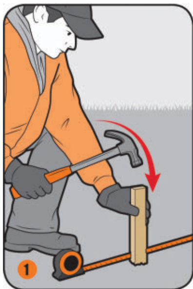
Mark off your fence layout with stakes and twine.
