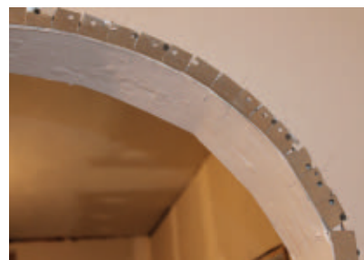
During the drywall phase, multiple sequential cuts were made in the corner bead so it would bend around the curve of the archway.
