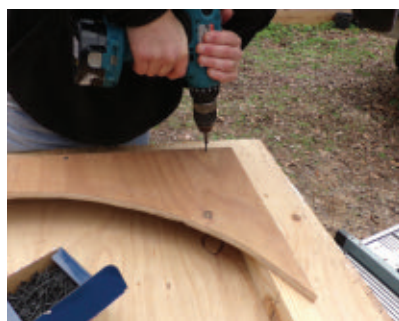
Fasten the panels with blocking between them.
