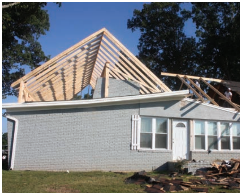
Ever wondered how a house changes hats? In this case, the contractors essentially built a new roof on top of the old one.
