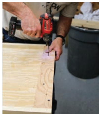
Attach the French cleat, as well as the side pieces that enclose the edges of the frame and hide the cleat.
