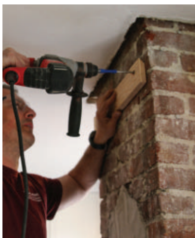
Mount the cleat to the wall.
