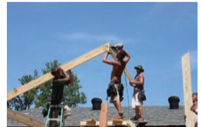
Roofing requires multiple workers to lift heavy materials and make proper connections in all the right spots.
