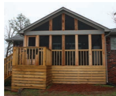
Here's the completed porch roof addition.
