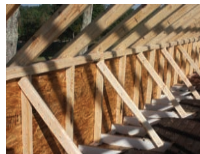
This knee-wall was constructed to raise the eave of the new roof and give the home a taller, grander design.
