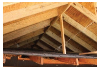
Shown is the new rafter system of the porch.
