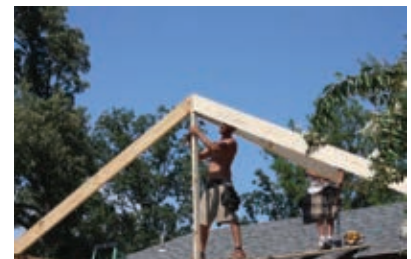
Temporary support braces are used to keep framing components in place while the roof-build continues.
