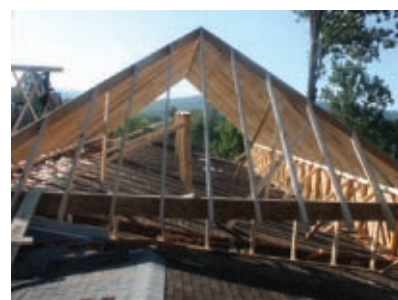
The old shingles are visible inside the framing of the new roof.
