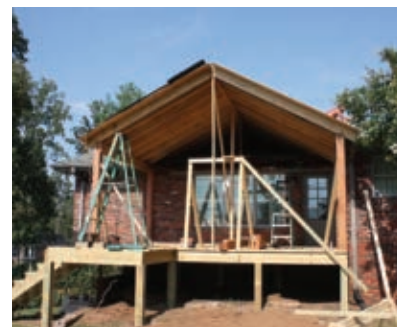
The roof is erected over a deck that will be screened as an outdoor living area.
