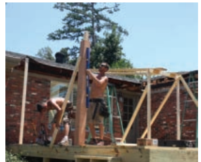
Some roof projects involve new additions to an existing roof. In this case the homeowners wanted a covered porch added to the rear of their house.
