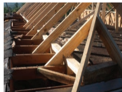
When necessary to tie the new rafters into the house framing, the workers cut into the old roof to make the secure connections.
