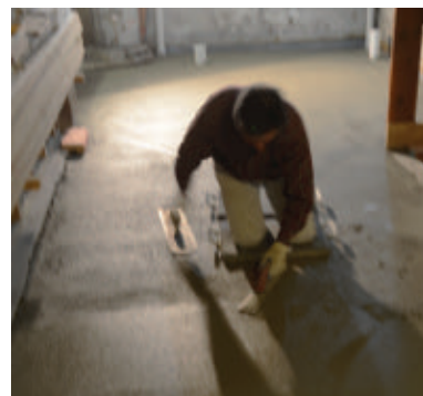
I could float the concrete floor, but could not float it well. That is a pro craftsman at work..
