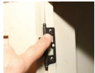
Remove the screw and clean out the damaged hole.
