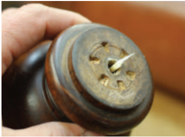
Break or cut the strips flush with the wood surface.
