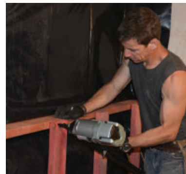
A 6-mil plastic vapor barrier fastened between the framing and foundation is effective, inexpensive and easy to install. Check local codes for the barrier that works where you live.
