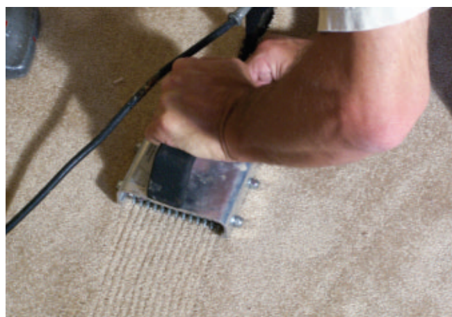
To join a seam, use a heat-bond iron and hot-glue seaming tape.
