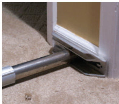
Position the foot of a carpet stretcher against solid wall framing.
