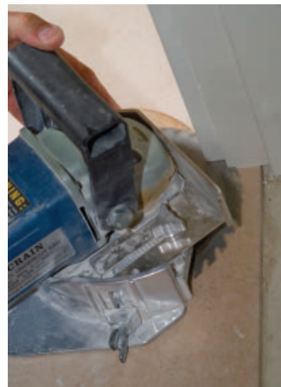
An undercut saw trims casings and door jambs very close to the floor so the sheet vinyl can tuck underneath.
