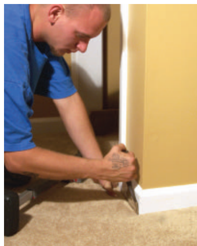
Tuck the carpet between the wall and the tack strip.
