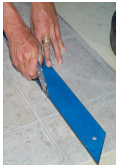
Use a straight edge and a sharp knife to make the initial rough cuts.
