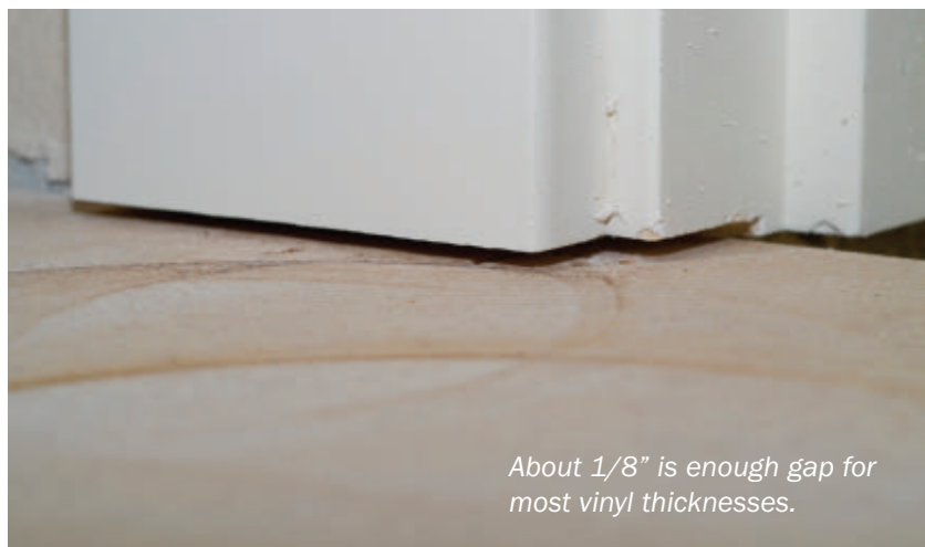
An undercut saw trims casings and door jambs very close to the floor so the sheet vinyl can tuck underneath.
