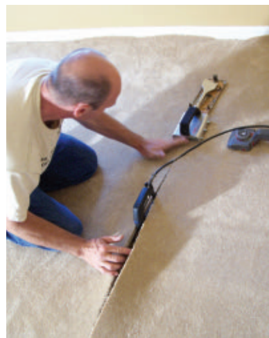
To join a seam, use a heat-bond iron and hot-glue seaming tape.
