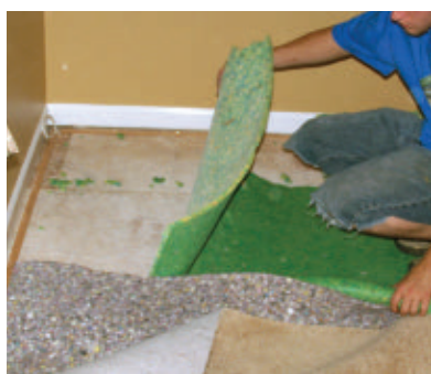
Tack strips and carpet padding are the first items to install.
