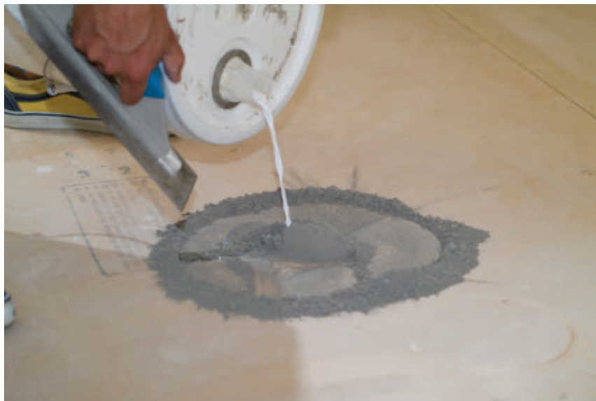
Mixing filler compounds right on the floor saves time and cleanup trouble.
