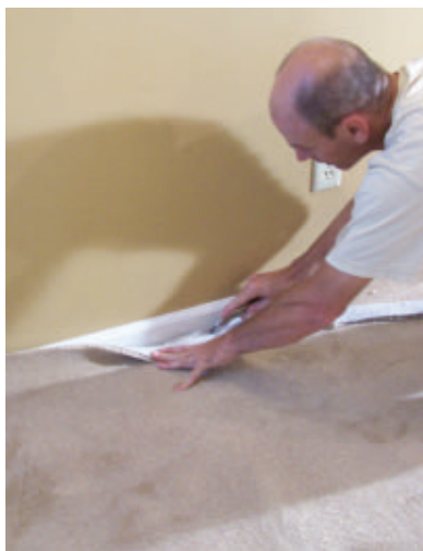
Proceed down the wall between the installed corners, anchoring the carpet and trimming the excess.
