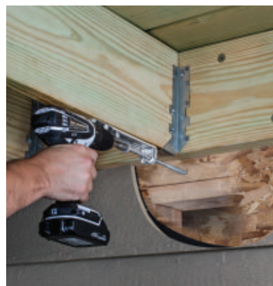
The DTT1Z deck tension-tie from Simpson Strong-Tie satisfies the latest deck ledger code requirements.
