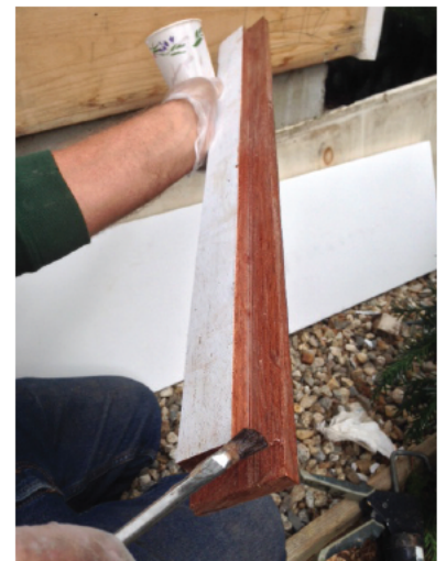
Cut the wood patch on a table saw and seal all edges.
