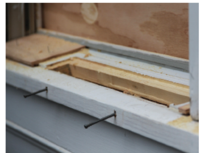
Shown here is the completed cut-out.
