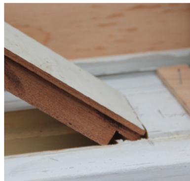
The patch should fit snugly as into the recess.
