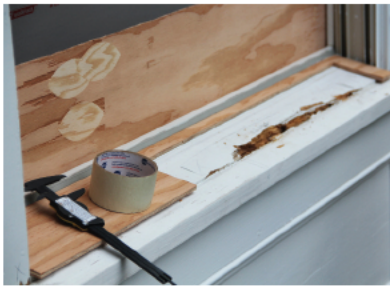
Surround the damaged area with wood strips to serve as a router guide.
