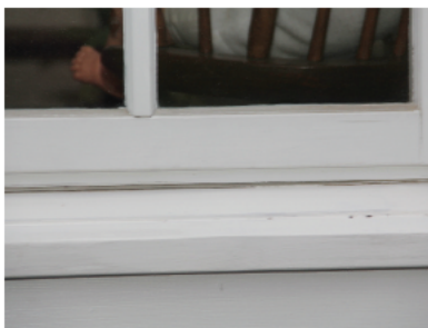
Finish the job by applying new caulk/sealant and a coat of fresh primer and paint.
