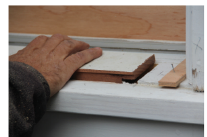
Test-fit the patch and make adjustments as necessary.
