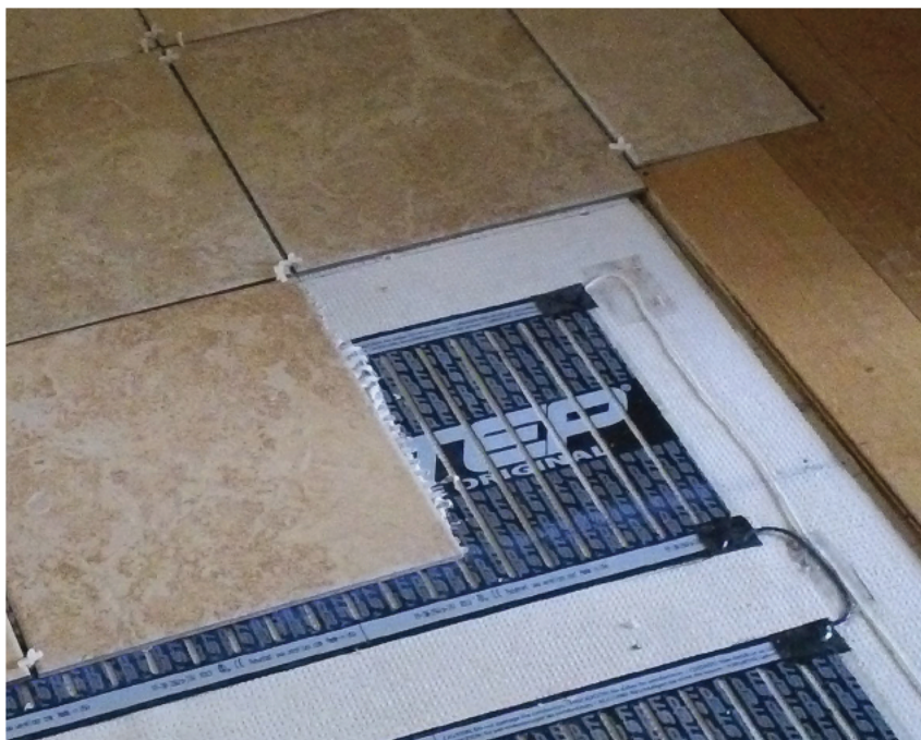
Radiant heat systems can warm cold tile floors. Photo courtesy STEP Warmfloor.
