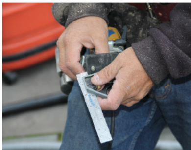
Set the depth of the router bit to create a stepped patch to fit into the window sill.
