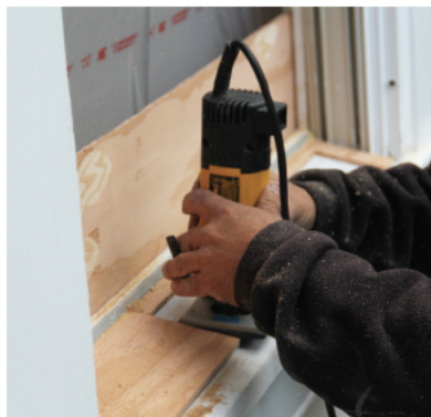
Carefully rout out the old wood.
