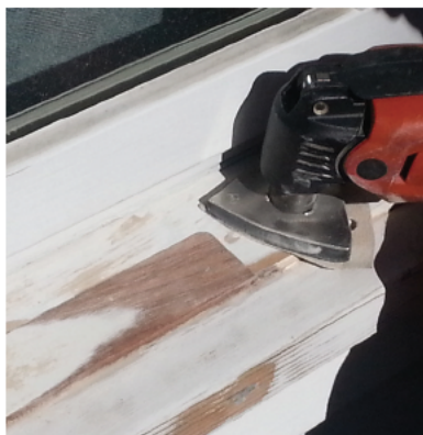
Sand the patch flush.
