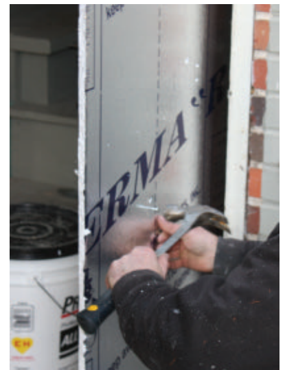
The foam sheets should be nailed to the wall studs.
