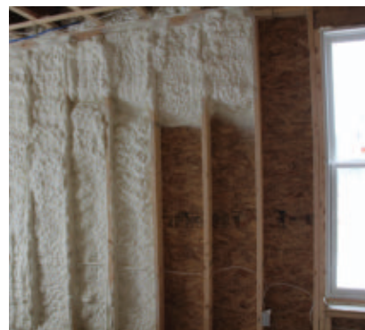
Exterior walls cavities were filled with spray foam insulation.
