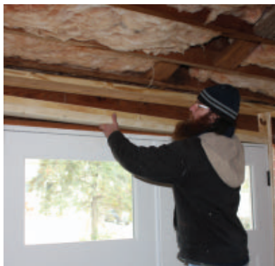
We installed the nonstructural 4x4 header.
