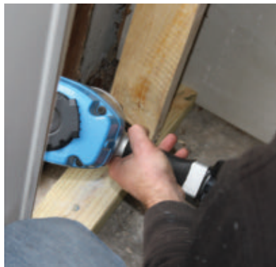
Toe-nail the studs in place at the top and bottom.
