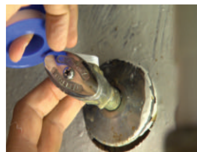
Apply Teflon tape to seal all thread-ed supply-line connections.
