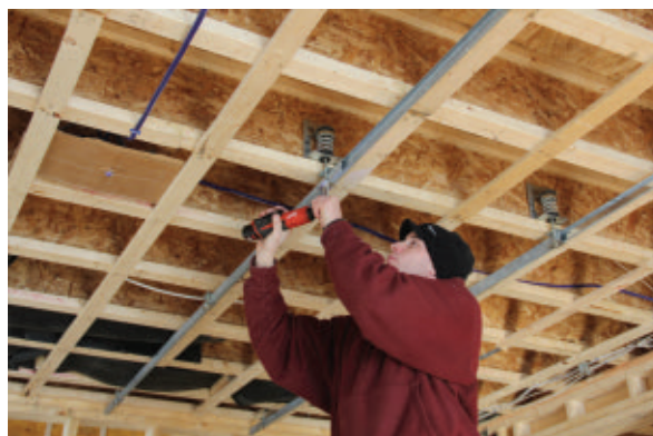
The ICW hangers can be installed 48 inches apart
