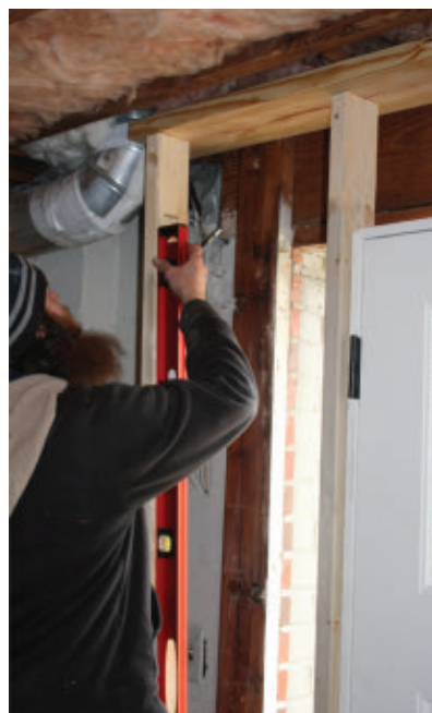
Make sure the studs are installed square, plumb and true and that the boards are straight and not bowed.
