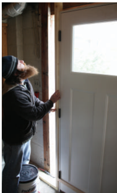
Install studs cut to fit between the sill and top plate, framing the sides of the rough opening.
