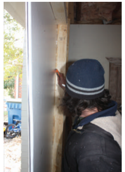
Use a utility knife to cut the foam sheet to fit the wall.
