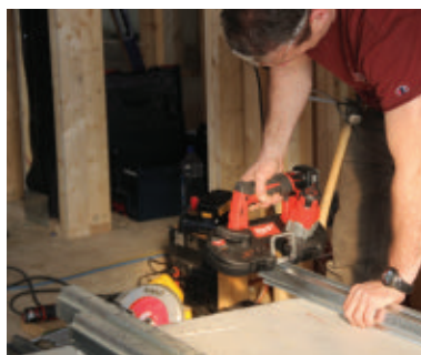
A band saw can be used to cut resilient channel to length without distorting its shape.
