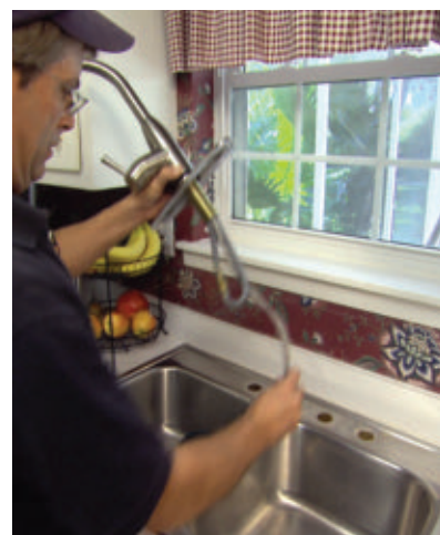
Feed the fixture through the mounting holes of the sink.
