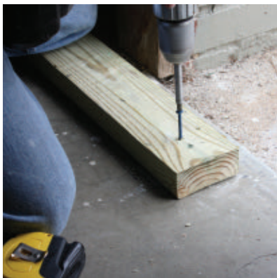
Anchor the wall's sill plate to the slab with concrete screws.
