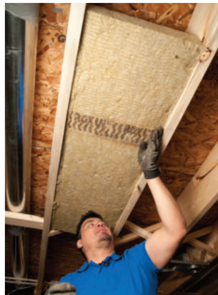
The batts compress to friction-fit between framing members for easy installation that requires no fasteners.
