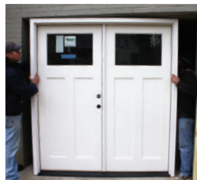
For this project we were able to position the new door and build the rough opening around it.
