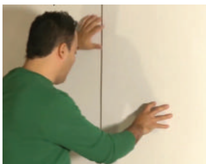
Further enhance the sound-dampening properties by installing a second layer of drywall, orienting the panels at right angles to the first layer. Finish the installation by sealing all seams with acoustical caulk.
