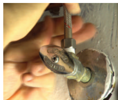
Reconnect the supply lines.
