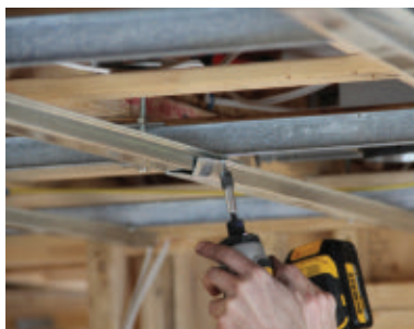
Screw the resilient channel into the 16-gauge steel, overlapping the ends to join separate segments.
