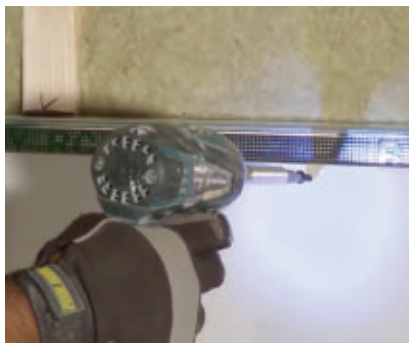
Screw drywall panels into the resilient channels between the studs to de-couple the wallboard from the framing.
