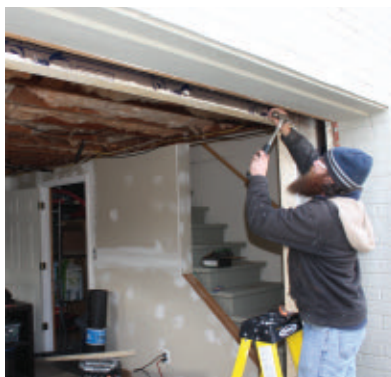
Rigid foam sheets helps to insulate the wall.
