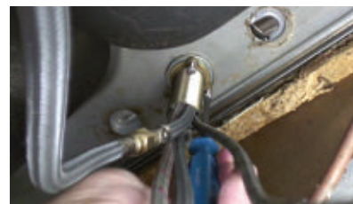
In this case, the new faucet runs all lines through a central location. Fasten all necessary screws, nuts or other hardware to securely mount the faucet to the sink.
