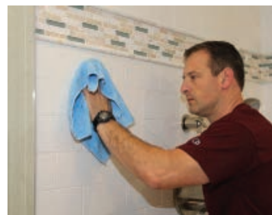
Clean the tile and grout thoroughly.
