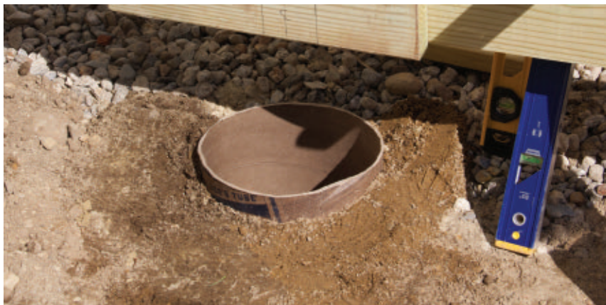
Tube-shaped cardboard forms can be cut to length and placed in the holes to pour the concrete footings.
