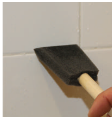
Use the the narrow tip to apply sealer to the grout lines.
