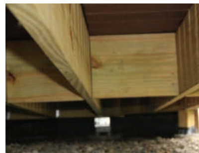
Small sections of joist material can be installed between the joists as mid-span blocking to help prevent deck bounce and strengthen through-the-deck rail post attachments.
