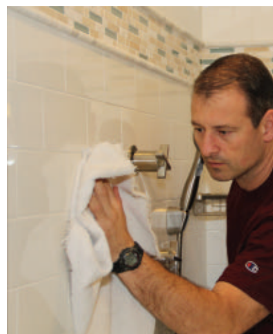
Allow to dry according to the manufacturer's instructions before applying second coat. Wipe away excess with a clean towel.
