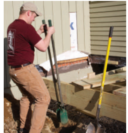
We dig concrete footings to support all deck posts.
