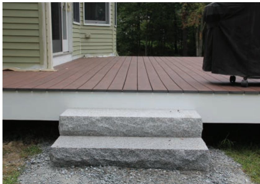
Granite steps provide access to the finished deck.
