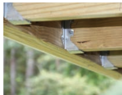
Use metal joist hangers to connect all joist ends.
