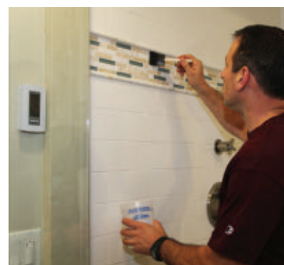
Apply sealer to the tile first using a foam brush.
