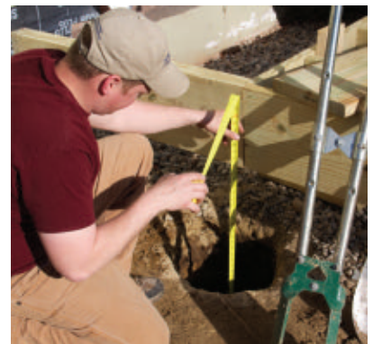
The depth of the deck footings will be determined by your local frost line and building codes.
