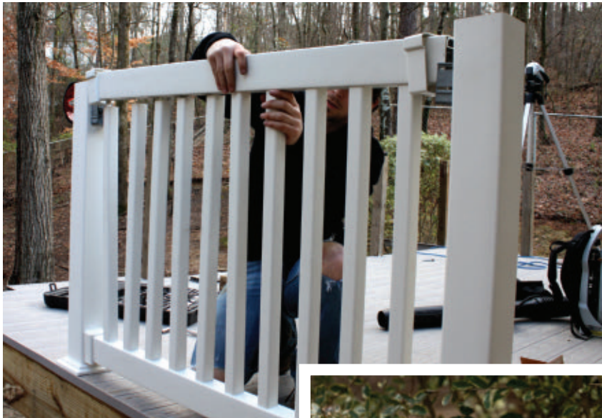
The top rail mounts over the balusters, followed by a rail cover for a comfortable hand grip.
