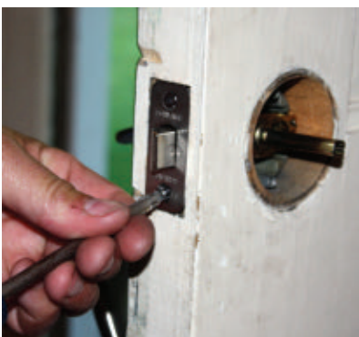
The faceplates install simply, using just two screws each.
