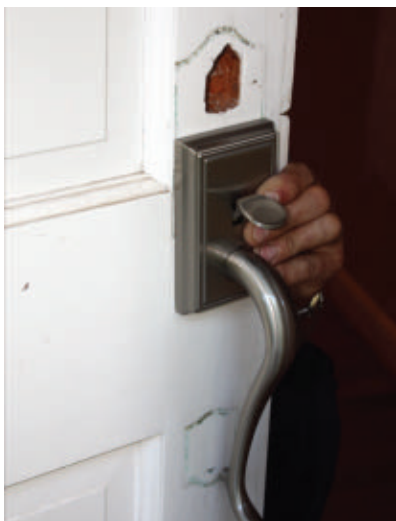
Test-fitting the new handle ensured that the existing knob hole was cut with the appropriate diameter.
