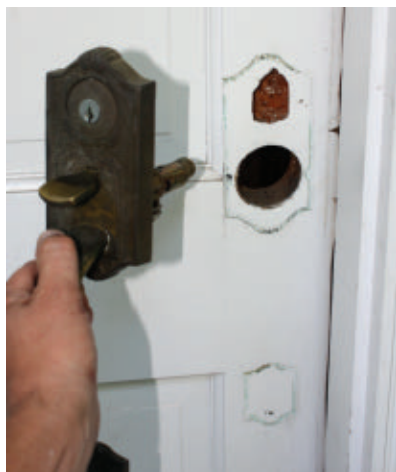
The old door handle had an integrated key, which left an ugly key hole in the door surface that we would have to fill and paint.
