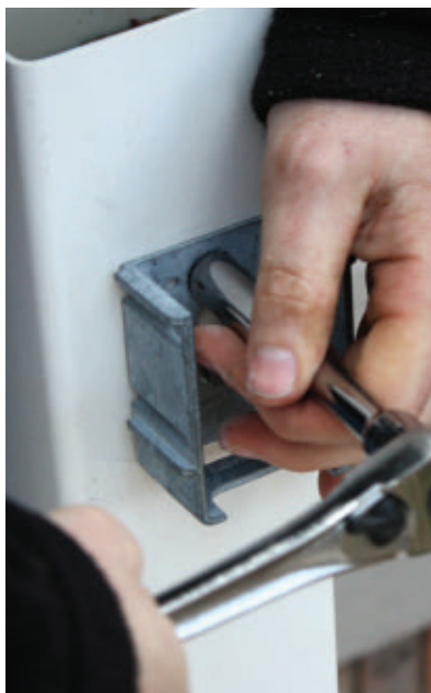
Each deck rail is supported by two metal mounting brackets that are bolted to the center of the posts.
