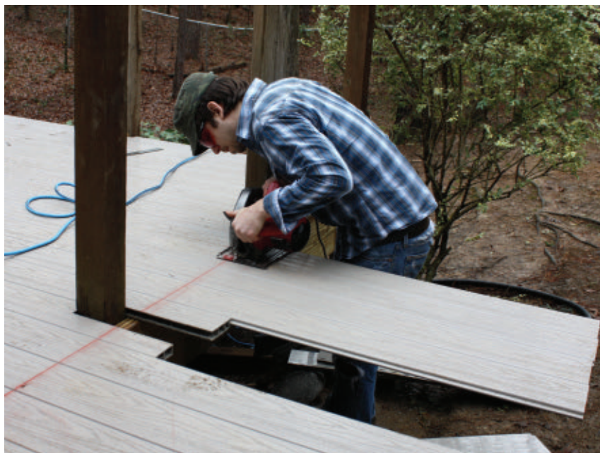
We ran the deck boards long and cut them all at once after installation was complete.
