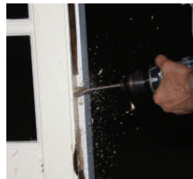
We used a spade bit to bore the holes for the bolt and strike plate.
