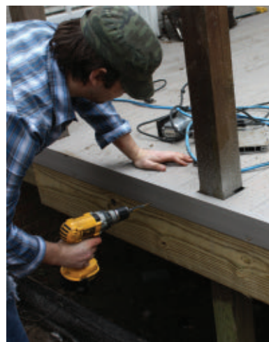
The L-shaped trim piece at the far end of the decking provides a finished look to the edges of the deck.
