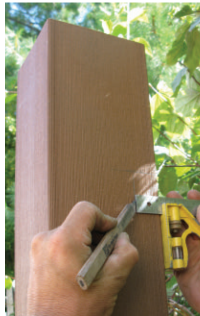
Mark the post height, mark the rail location and install the rail bracket. Or, use cleats as in a wood fence.
