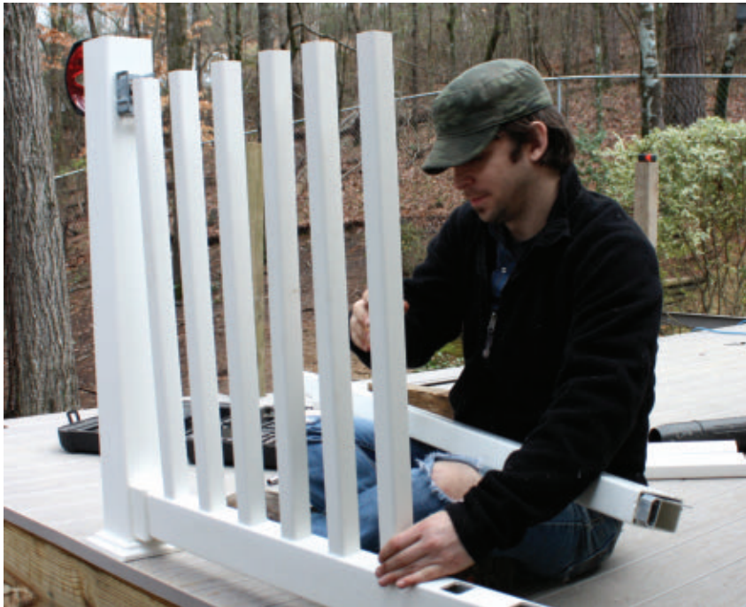
The balusters simply slip into the routed holes of the rails.
