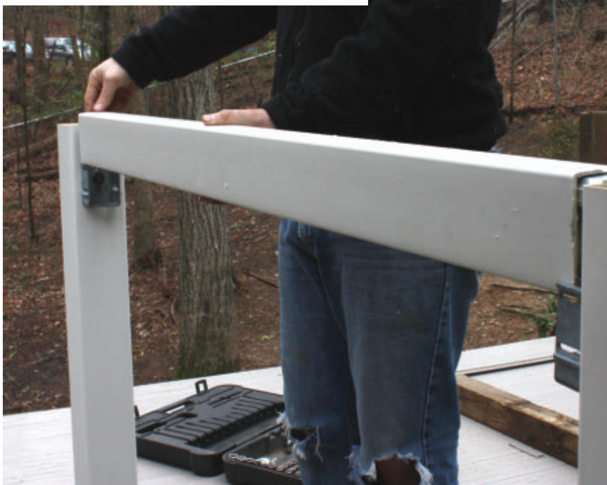
The PVC deck railing begins with the installation of post covers that slip right over the existing 4x4's.
