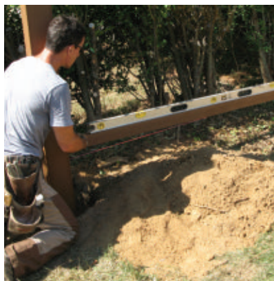
Set the rail layout on the high side then level over to the low side, mark the post and set the bracket.
