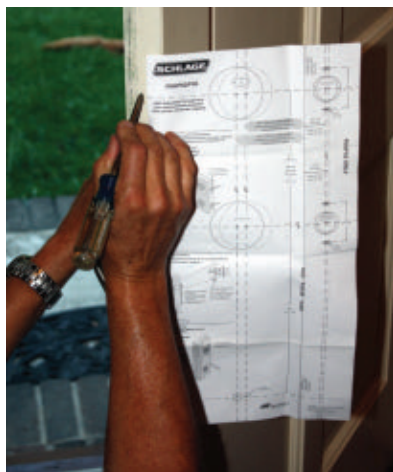
Schlage includes a paper template to help locate the holes for the door hardware.
