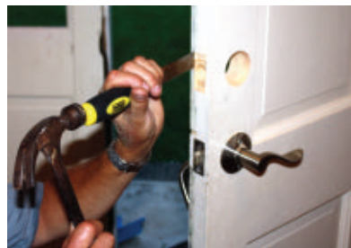
A wood chisel and hammer are required to cut the mortises for the faceplates.
