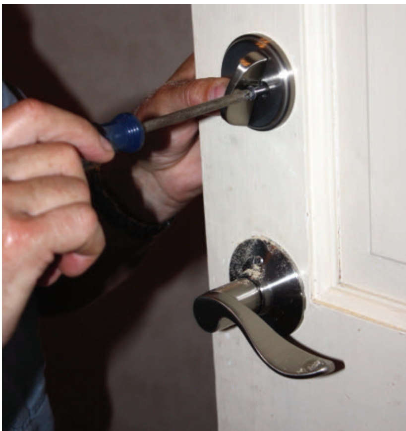
Fastening the deadbolt assembly is the last step in installing the new handle-set.
