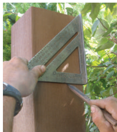
Mark the post height, mark the rail location and install the rail bracket. Or, use cleats as in a wood fence.
