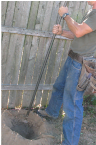
Tamp the soft earth with the blunt end of a digging bar.
