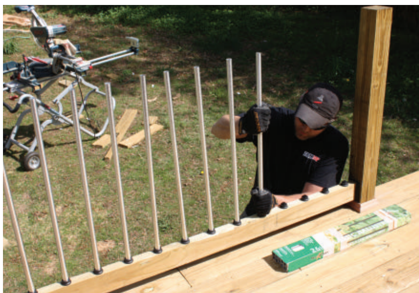
Slide the aluminum balusters onto the rubber baluster connectors.
