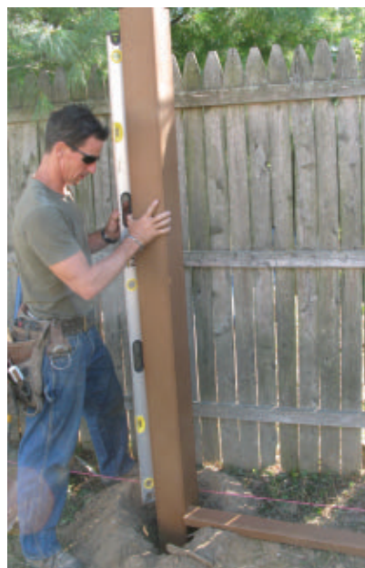
Set the post in the hole. Use rail stock as a gauge-stick and plumb both faces of the post.
