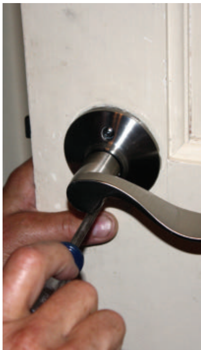
Two bolts are all that's required to install the interior handle.
