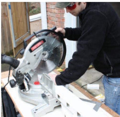
The PVC Rails, the Aluminum P-channel Inserts and the Rail Covers are all cut to length, according to your post layout. When cutting the rails, be sure to keep the routed holes in the rail spaced symmetrically (they accept the balusters).
