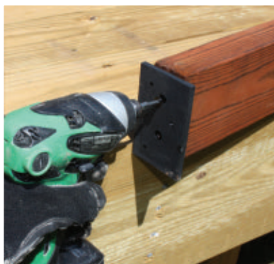
Screw on the plastic Railing Connector, and fasten the lower rail between the posts.
