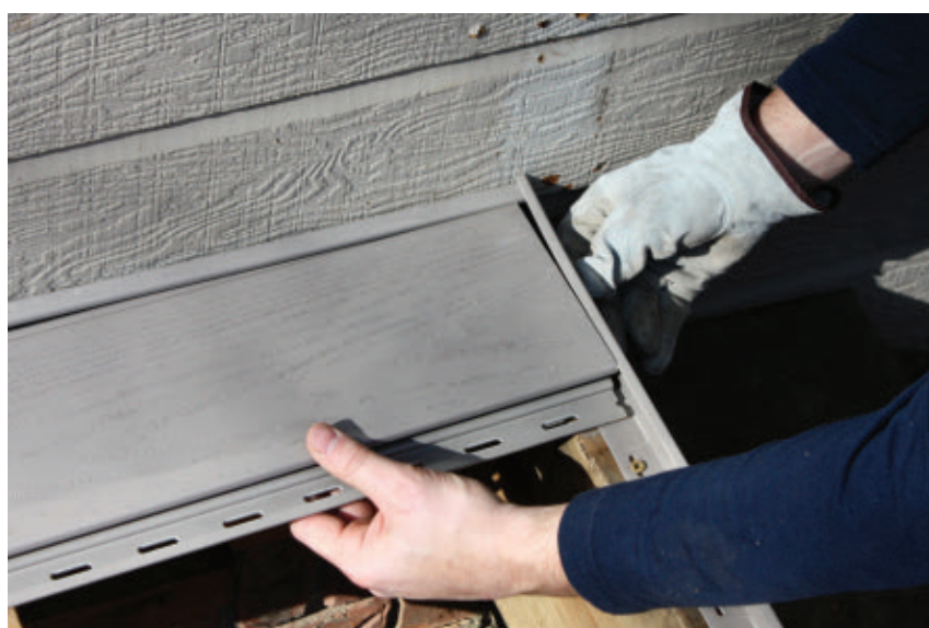
Installation begins with a starter strip fastened over the ledger board and an adjacent trim strip fastened to one of the rim joists, which conceals the ends of the deck boards.
