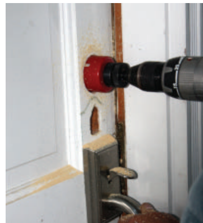
A hole-saw was necessary to cut a new hole for the deadbolt assembly.
