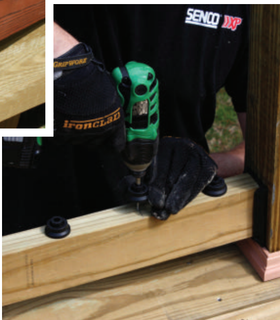
Attach the Designer Baluster Connectors on each mark.
