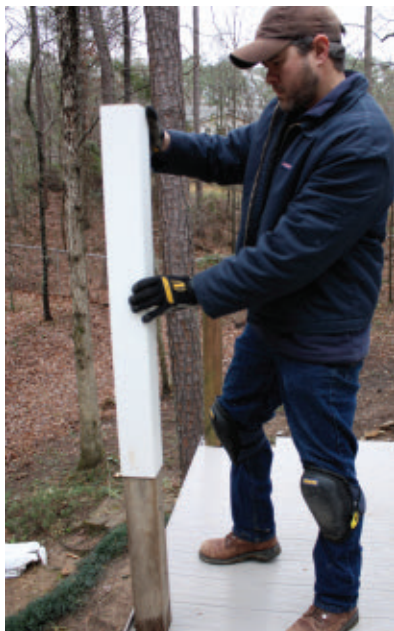
The PVC deck railing begins with the installation of post covers that slip right over the existing 4x4's.
