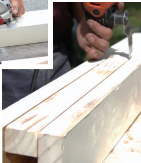
The notched cuts were started with a circular saw and completed with a multi-tool.
