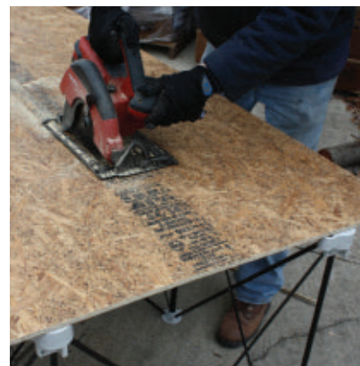
Installation requires a substrate of 7/16" or greater OSB or plywood.
