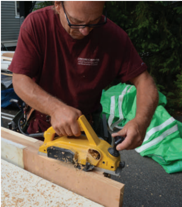
The repair and post are then planed together.
