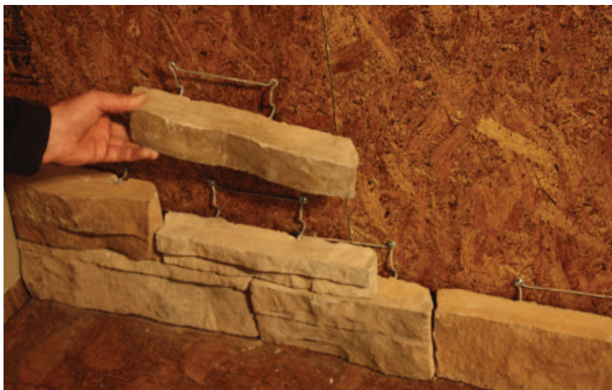
Stagger joints from row to row. Some stones are half the height of others and require two stones to be stacked together.
