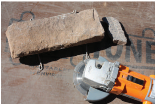
Cut the stones using a chop saw or a grinder with a diamond-grit blade.
