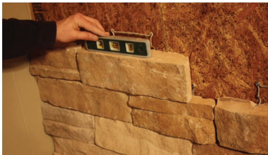
Check each stone for level.
