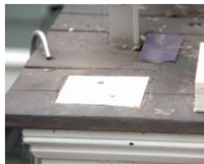
The porch decking is cut out and a PVC shim is installed beneath the post location.
