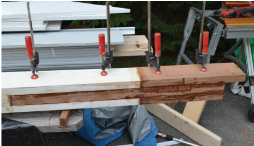
Additional cedar blocking was epoxied and clamped onto the keyed piece to extend and strengthen the post base.
