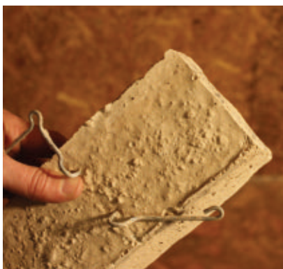
I bent the lower hooks out of the way to install the first stone.
