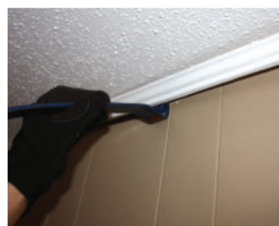
First step was to remove all molding and trim.
