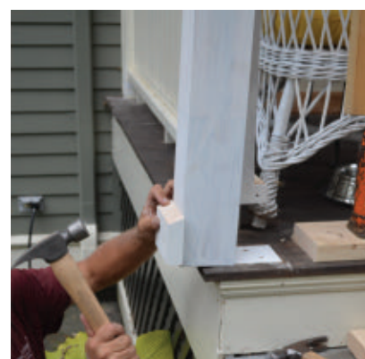
Lift the overhead structure slightly with the jack and install the repaired post.
