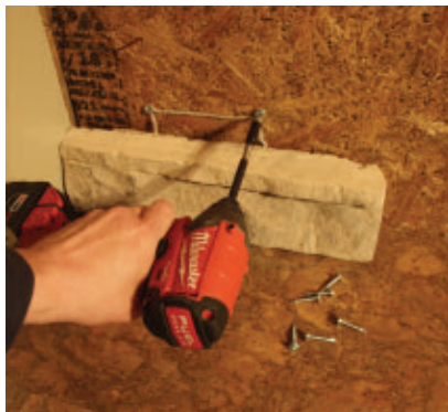
Each stone installs with two screws.
