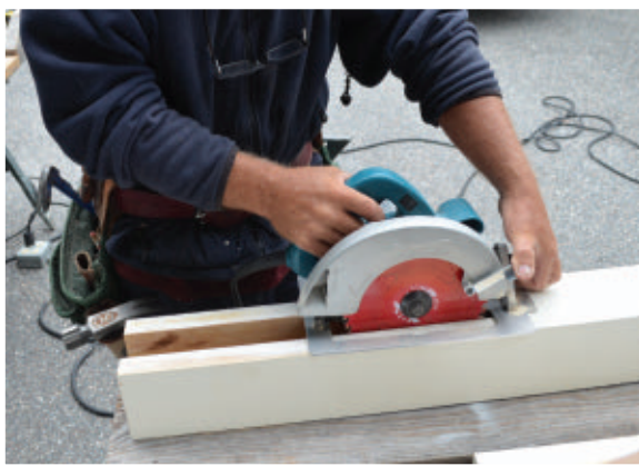
To avoid a weak hinge point where the new wood is spliced into the old, the post was cut above the rot to allow room for an interlocking stepped, keyed joint.
