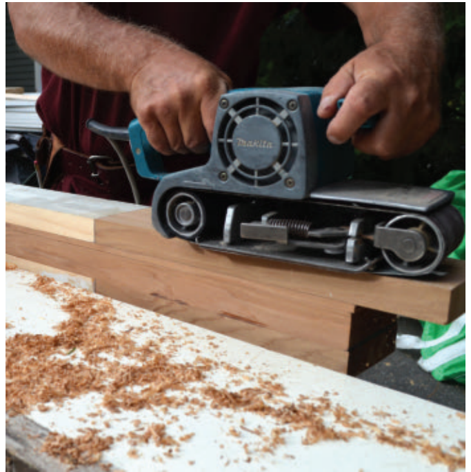
The joint is fine-tuned with a belt sander.
