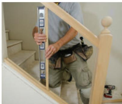
A scrap of material was used to test-fit a baluster, which allowed us to get the correct angle and lengths. Be sure to test the baluster pattern at both ends of the balustrade. A minor difference in knee-wall or rail-rake angle can affect the baluster length from one end to the other.
