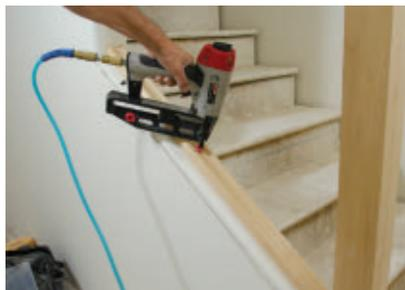
The shoe rail was nailed with 2-1/2" finish nails in the center of the knee wall. We often use a piece of scrap material as a pattern to test the angles and the lengths of the rails before cutting the rails. Unlike a lot of other material on the job, you usually don't have additional rail on the jobsite to cover for a bad cut.
