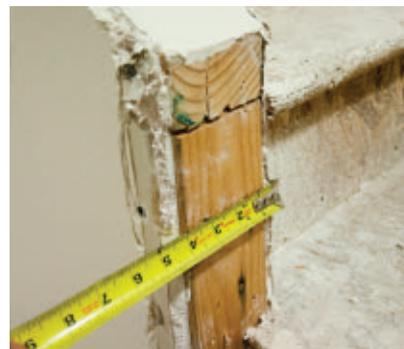
*After getting to bare framing at the end of the knee wall, we measured the thickness of the knee wall in several places to determine the width of our wall cap.*
