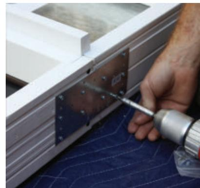
*For maximum rigidity, fill all holes in the metal plates with screws.*
