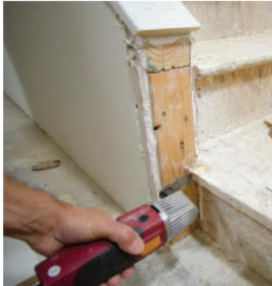
Cutting a notch in the nose of the landing made room for the vertical wall piece.
