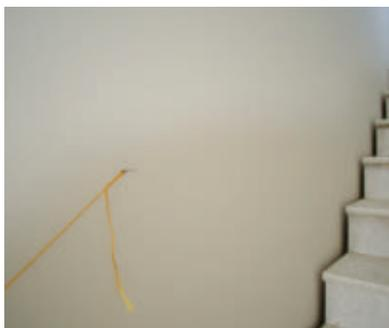
*One trick is to put a nail in the wall at the top-of-the-handrail mark and pull a string to the mark on the level as it is held plumb on the stair nosing at the bottom of the open rail run.*
