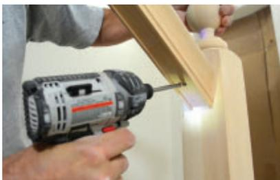
With top of the rail anchored, we returned to the tacked-in-place bottom of the rail and more solidly attached it to the newel post with a long screw through the plow and into the newel post.
