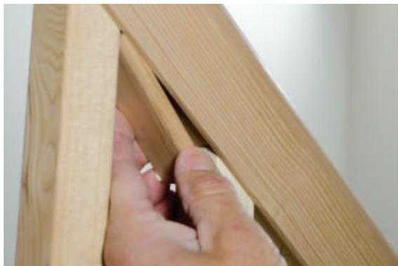
We held the fillets up flush with the bottom of the rail and marked where they overlapped the next baluster, then trimmed them to length. It's a good idea to number the backside of each fillet and put a matching number inside the plow where the fillet belongs on the rail.
