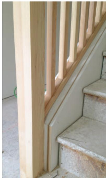
Notice that the stair skirt covers the drywall at the inside of the staircase and is fit to a 1/4" reveal on the knee wall cap.
