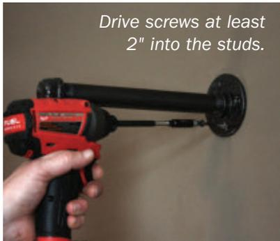
*Drive screws at least 2" into the studs.*
