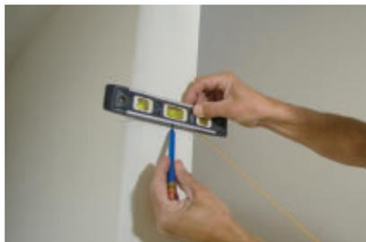
We used a torpedo level to transfer the handrail layout from the string to the center of the wall where the top of the handrail would terminate.
