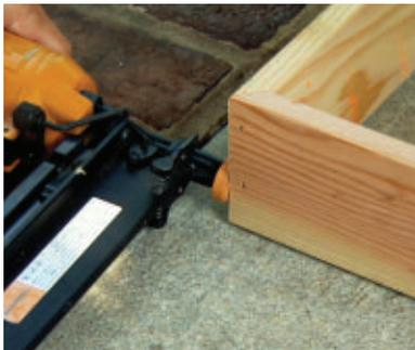
Fasten the the miters with brad nails driven in a cross pattern.
