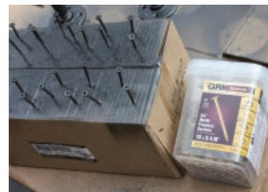
Paint the screw heads to match. I used #10 x 3-1/8" R4 Screws from GRK Fasteners.
