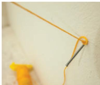
*In our case, the handrail layout line terminated in the wall so we put a finish nail at a very steep angle up into the wall to make an anchor point for the end of the handrail layout string.*
