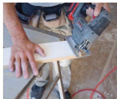
A jigsaw was used to cut the bevel at the top end of the wall because it had to match the drywall corner bead on each side. For most of our staircases this angle is about 37 degrees.
