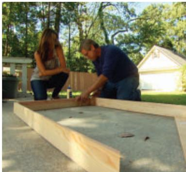
Assemble on a very flat surface to ensure tight joints. Use corner clamps if necessary.
