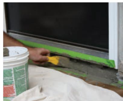
We completed the job with fresh mortar beneath the threshold.
