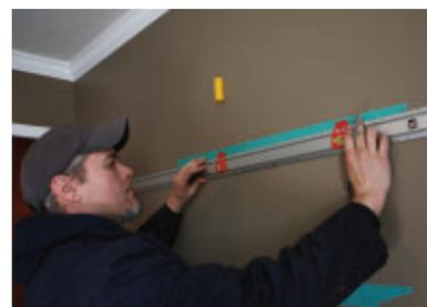
*Locate each pair of the brackets the same distance apart and perfectly level.*
