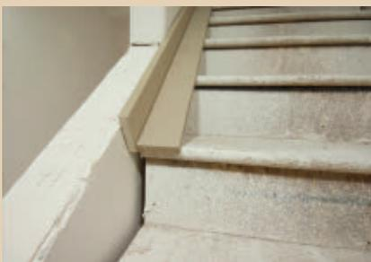
We made this jig of 1x4 by ripping the vertical piece so it matches the top of the knee wall framing plus the thickness of the wall cap.
