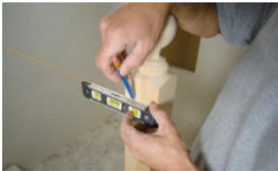
We stood the newel post in place at the end of the knee wall and used a torpedo level to mark where the handrail would intersect the newel post.
