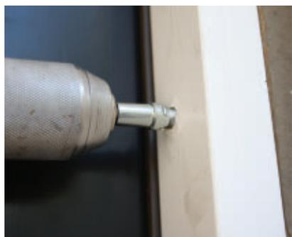
For this installation we used Top Star Shim Screws from GRK fasteners.
