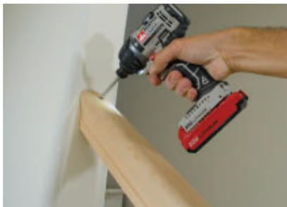
After fitting the handrail, we tacked it into the newel post at the bottom and counter-bored for a long screw where the rail meets the wall. Driving a long screw through the rail and into the framing is an important detail to make a strong connection.
