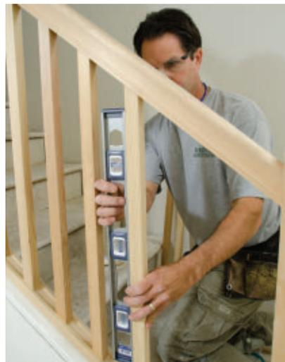
We used a 2' level to test each baluster at its location before gluing and nailing them into place.
