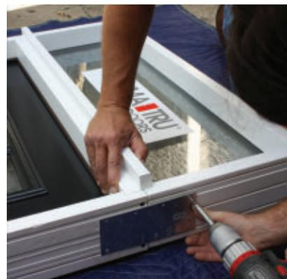
*The jambs are attached at the sides with metal hardware.*
