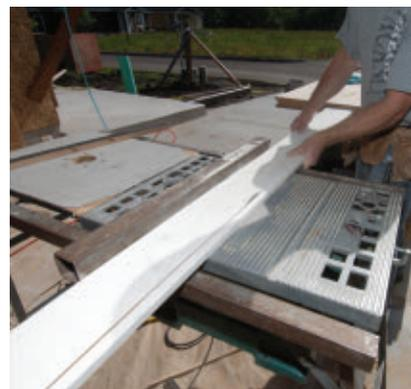
After taking a rough measurement for the length of the knee wall and the knee wall face, we ripped the wall cap material to width on the table saw and cleaned it up with a planer, sander and router.
