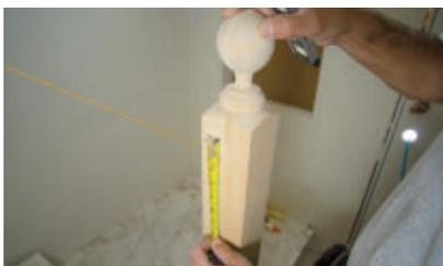
We measured from the mark on the newel post up to the desired intersection point (where we wanted the handrail to terminate), which indicated how much to cut off the base of the newel post.
