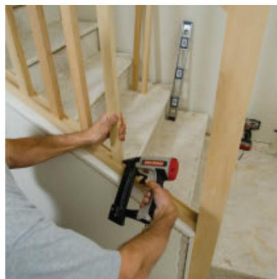
After gluing the top and bottom of the baluster and fitting them into the rails at the layout marks, we used 1-1/4" finish nails to toenail the balusters from the obtuse side.
