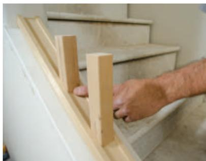
We used the end cuts from a few balusters to test the baluster layout by standing them in the shoe rail.
