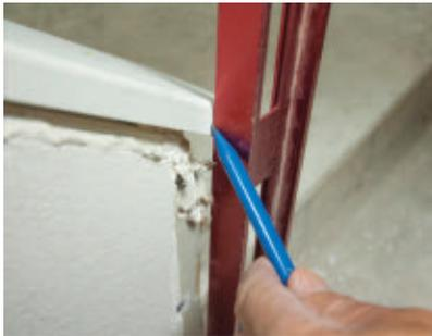
After fitting the wall cap to the vertical wall at the top end of the knee wall, we tacked it into place and used a level to mark where the bottom edge of the wall was plumb with the front face of the knee-wall framing.
