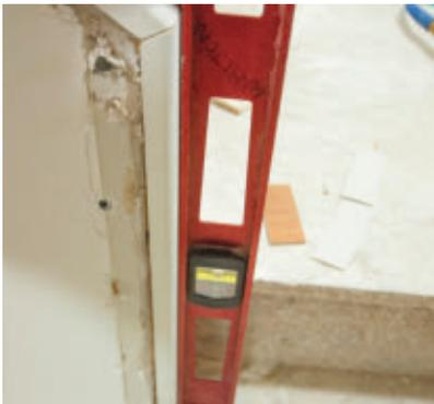
We cut the end of the wall to bisect the angle where the knee-wall face meets the wall cap. The cut is usually about 27 degrees. You can cut some scrap material to test the angles ahead of time.
