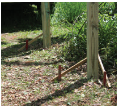
Brace the posts from each side to hold them in position while you pour the concrete footings.
