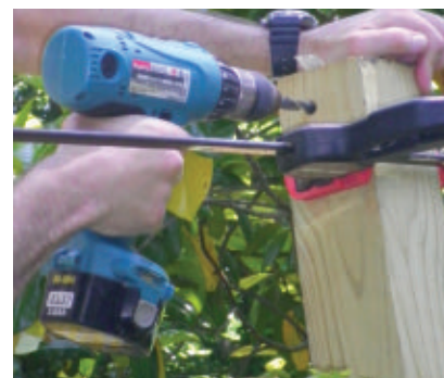
The band is fastened to the posts with 6" carriage bolts.
