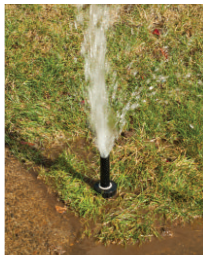
I started the sprinkler zone with the sprinkler nozzle removed from the riser to clear debris from the pipe.
