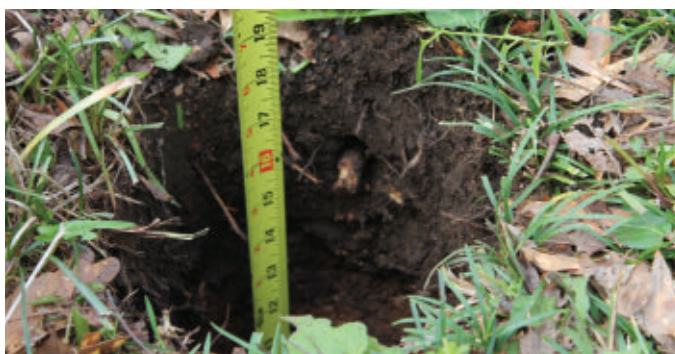
Calculate your measurements according to the center point of the post holes.
