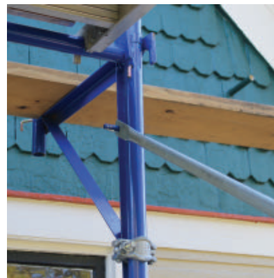
End brackets hook and bolt onto the scaffolding frame to extend the work area.
