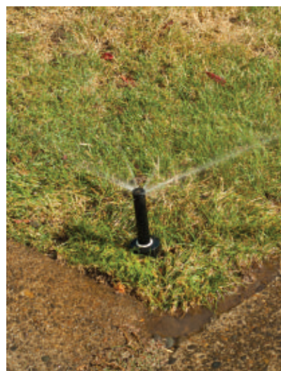
After replacing the nozzle, I adjusted the sprinkler and tested it for the running time of the zone. EHT
