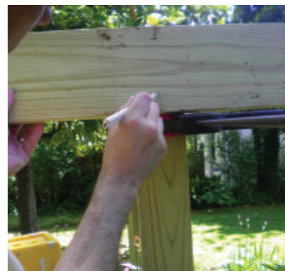
Mark corresponding bolt holes on both the posts and the 2x6 band.
