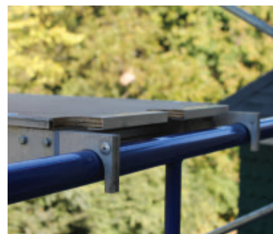
The walk boards hook over the tubular frames with a firm connection that prevents slippage underfoot.
