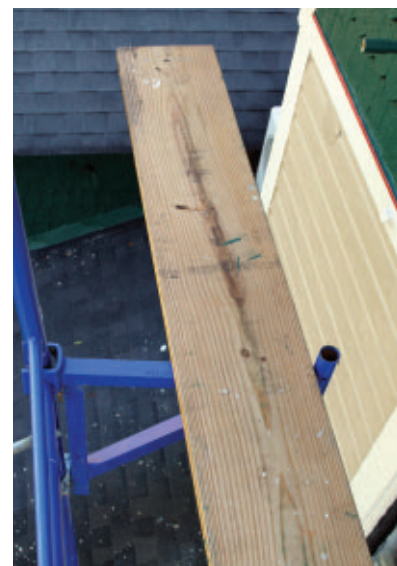
To handle extra materials, equip the brackets with boards to expand the work surface.
