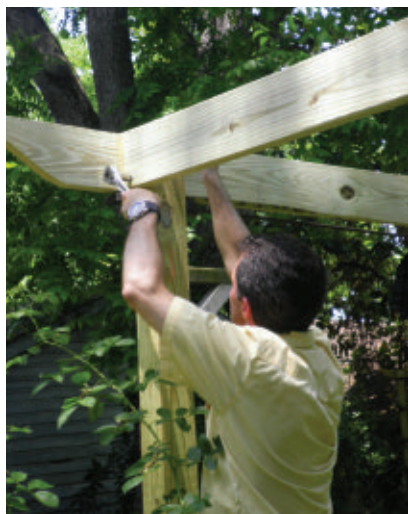
Tighten all carriage-bolt connections with a wrench and socket set.
