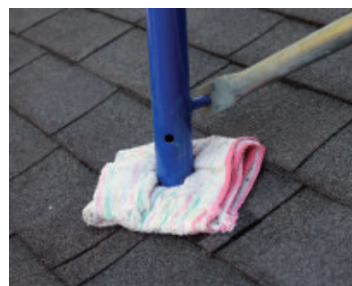
When positioning on a roof, it's smart to protect the finished surface from damage by the scaffolding.
