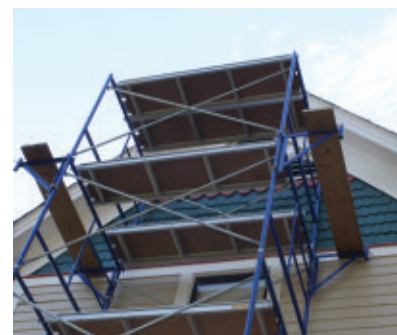
Side brackets accomplish the same work-surface extension on the sides of the scaffolding.
