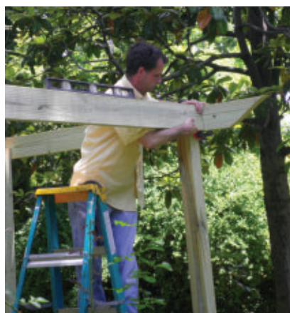
With the band complete, the vertical top boards can be toe-nailed 16" on center.
