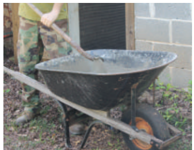
Ready-mix concrete is easy to mix with water in a wheelbarrow using a shovel.
