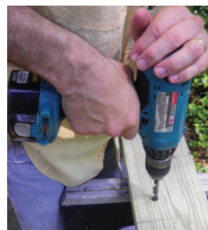
Drill matching pilot holes in the posts and the band.
