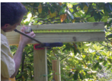
Install the 2x6 band, ensuring an equal overhang on both opposing face boards.
