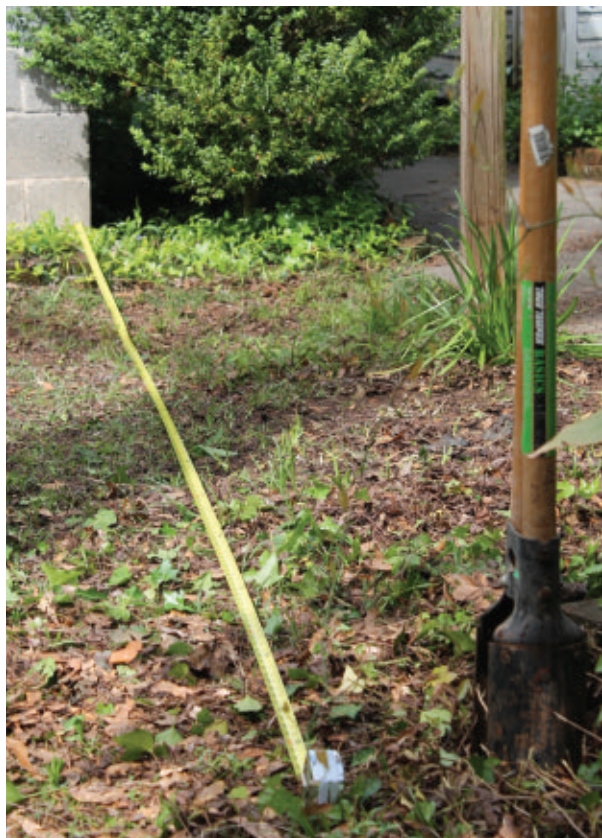
Carefully lay out your post locations in relation to any nearby structure.
