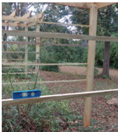
The horizontal runners were ripped from 1x lumber into inch-thick strips and finish-nailed up the sides of the arbor every 12".
