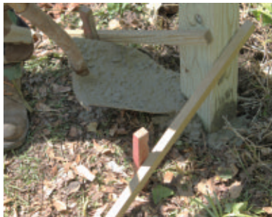
Roughly 50 lbs. of concrete anchors the posts.
