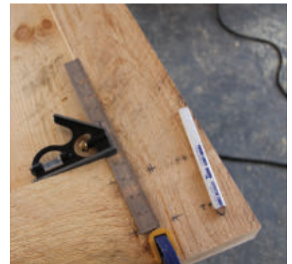
Check for square at every joint before fastening.
