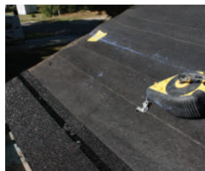
Chalk lines can help guide the layout.
