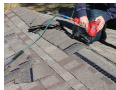
Fasten Ridge shingles over the ridgeline with two nails each.
