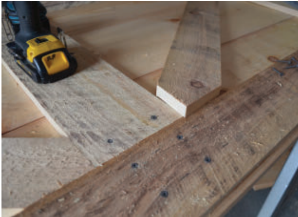
The diagonal braces are critical components to prevent the door from racking and sagging.
