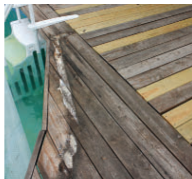
The rebuilt deck with old and new boards. Note the rot on the pool edges, these boards haven't been replaced yet.
