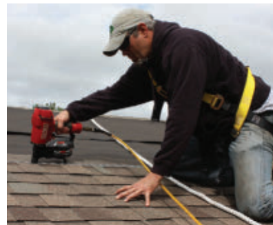
A fall-restraint safety harness should be used when working on the roof.
