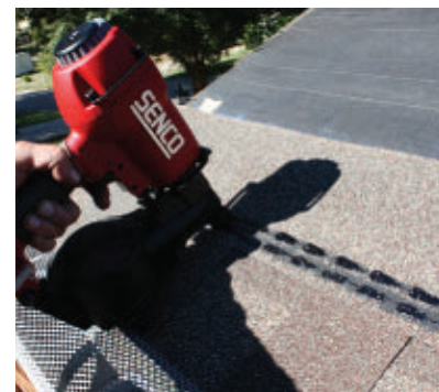
Begin the first course with a full shingle at the lower left corner of the rake.
