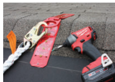
I attached the 3M fall-restraint harness to the roof ridge with 10 heavy-duty screws.
