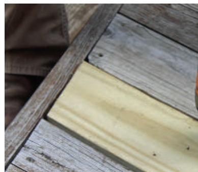
New boards are installed with quality exterior deck screws.
