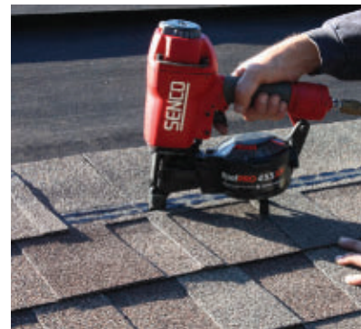
The Senco RoofPro 455XP is handy new roofing nailer that saved lots of time on this job.
