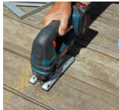
A saber saw is used to make the cut. The Bosch cordless saw is ideal for the job.
