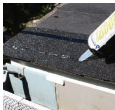
I applied Through the Roof roofing sealant above and below the starter strip.
