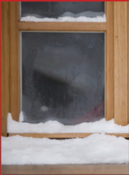
In freezing temperatures
