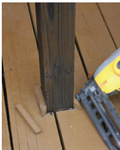
Trim boards are then installed using a cordless finish nailer and stainless steel finish nails.
