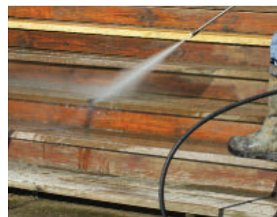
The deck and steps are lightly power-washed.
