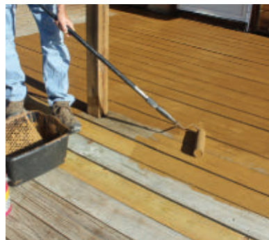
The Superdeck Deck & Dock is rolled onto the cleaned, dry surfaces.
