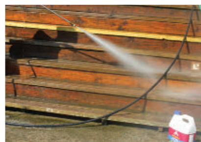
The deck is brush-scrubbed and power-washed.
