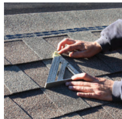
I marked a Speed Square with tape to spot-check the shingle exposure.
