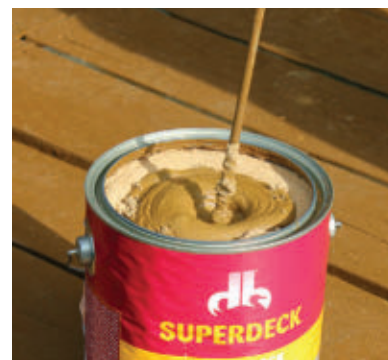
The additive must be thoroughly mixed into the coating.
