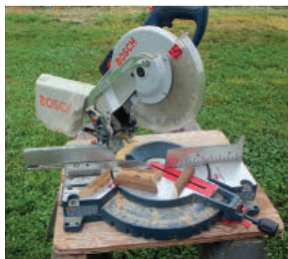
Trim boards are first routed to create a rounded edge, then cut to 45 degree angles to fit around awning posts. The Bosch cordless miter saw makes the on-site work easy.
