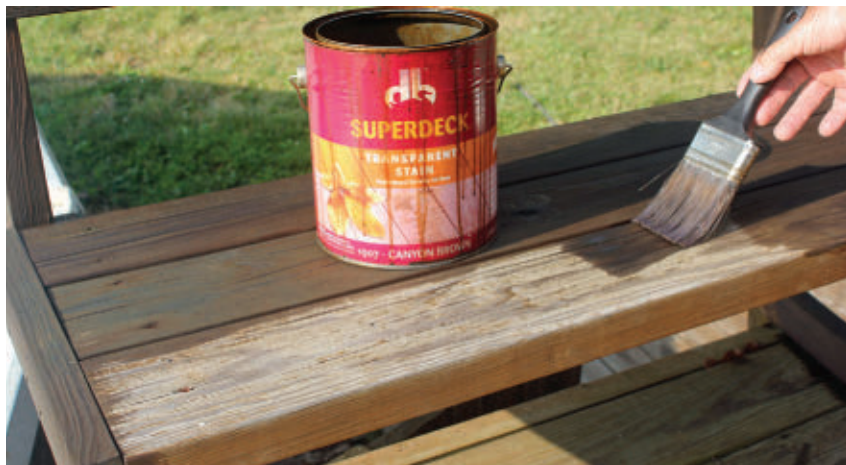
Pool railing and benches are stained using Superdeck Transparent stain. Note the benches were stained prior to deck coating. The railings were removed, stained and then reinstalled.
