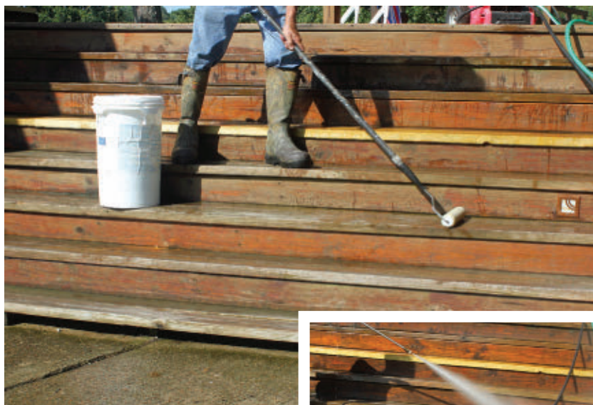
The diluted cleaner is applied with a roller.
