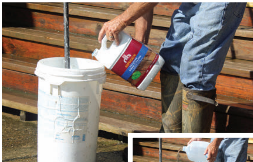
Super Deck Exterior Cleaner concentrate is used to clean the wet areas.
