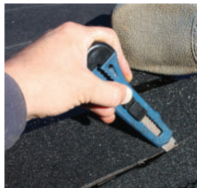
My starter strip was too wide for the underlying shingle tabs, so I trimmed to fit.
