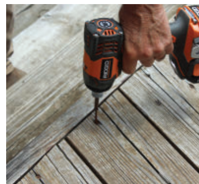
Old screws are removed using an impact driver. Go slowly or you may strip out heads and have a real problem.
