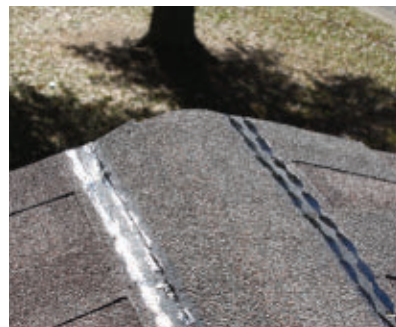
We installed shingles all the way to the ridge line then trimmed the excess at the top.
