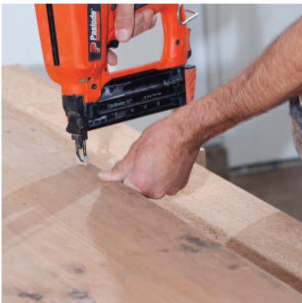
Tack the plywood to the runners in a few places to keep the edges lined up.
