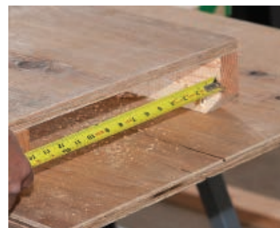
Measure the space between the two table supports and cut wing boards that will fit underneath with about 1/2" of room.
