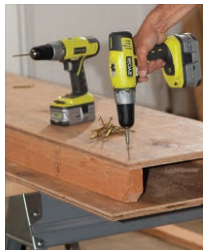
Pre-drill and screw the plywood to the runners with drywall screws.
