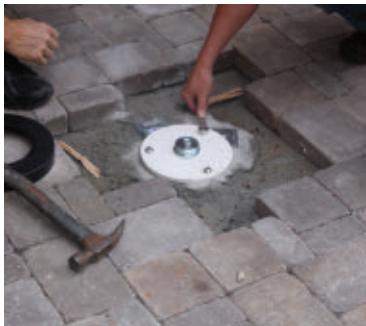
Install the base plate.
