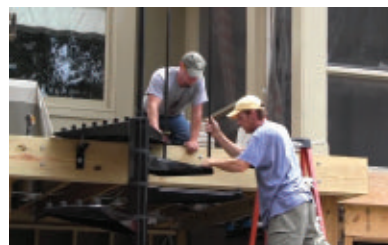
The next step is baluster installation.
