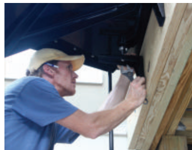
Attach the landing to the finished floor with the included hardware.
