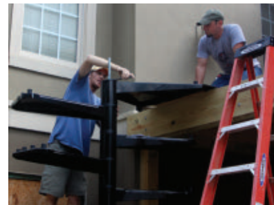
The staircase shown has a mezzanine landing.
