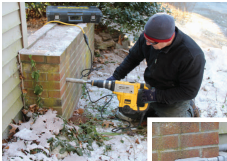
A rotary hammer bores through the brick to route the electrical supply.
