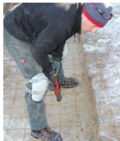
The mesh is cut to fit the curve of the walkway.
