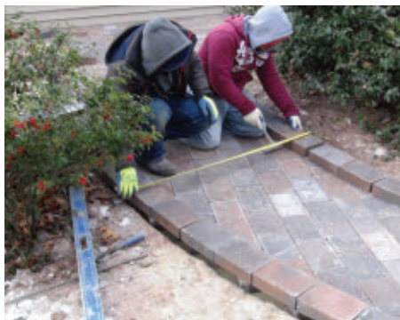
Border pavers help to give the walkway a finished look.
