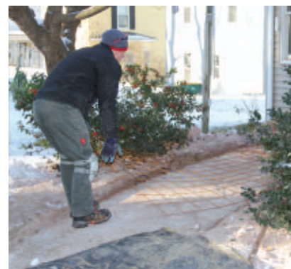
The mesh is placed over the compacted sub-base, and sand will cover both the mesh and heating cable.
