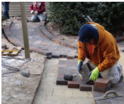
The paver stones are carefully laid onto the sand bed.
