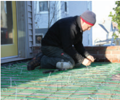
The cable is secured to the mesh with tie-wraps. I drilled through the brick wall in the photo for the electrical supply line.
