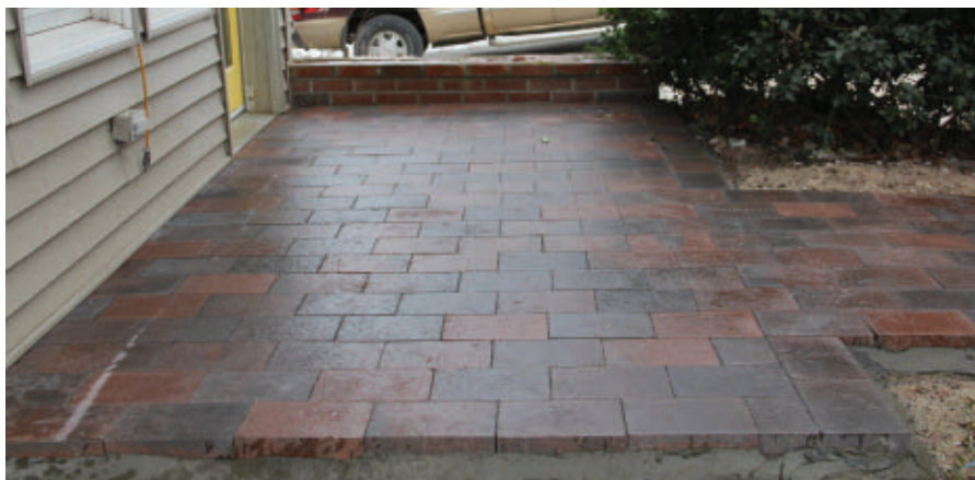
Here's is the completed new landing, after polymeric sand has been swept into the paver joints and the surface has been rinsed.
