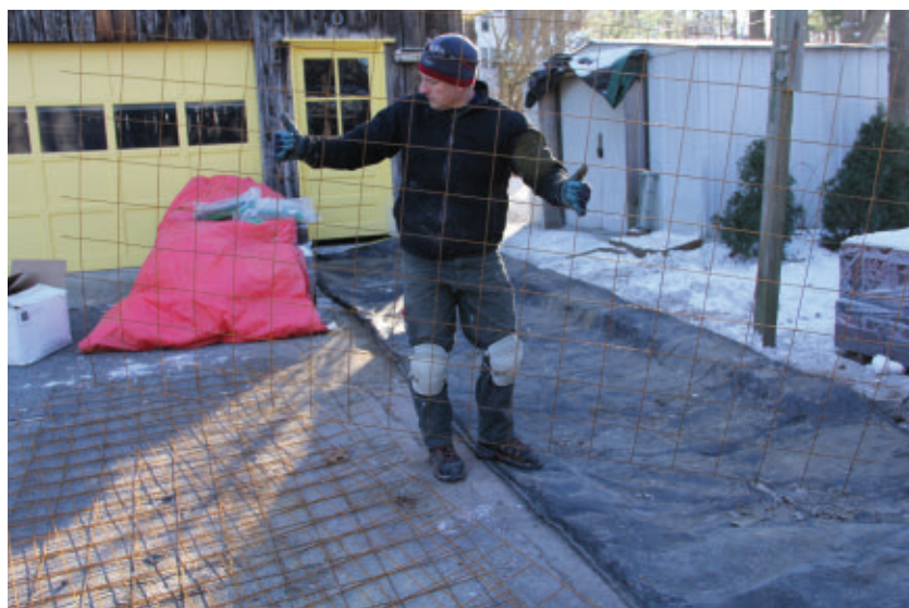
Wire mesh is used to anchor the heating cable.
