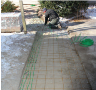
The green heating cable is routed along the wire mesh.
