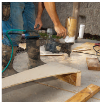
The door transom was traced on a sheet of OSB to copy the shape.
