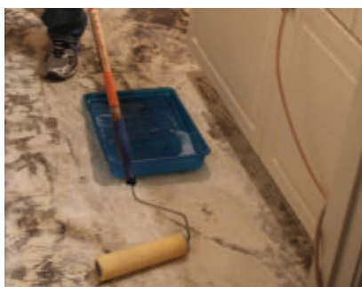
Multipurpose Floor Primer will help ensure a firm glue bond with the subfloor. I applied the primer with a paint roller.
