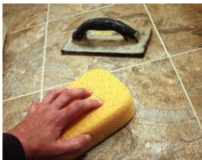
Use a sponge and plenty of clean water to clean up excess grout as your work.
