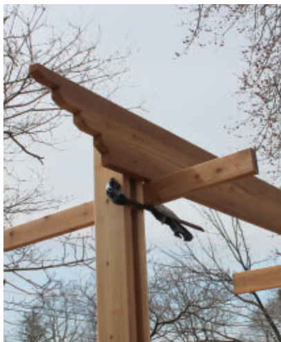
Clamps and cleats make installing girders much easier and safer.
