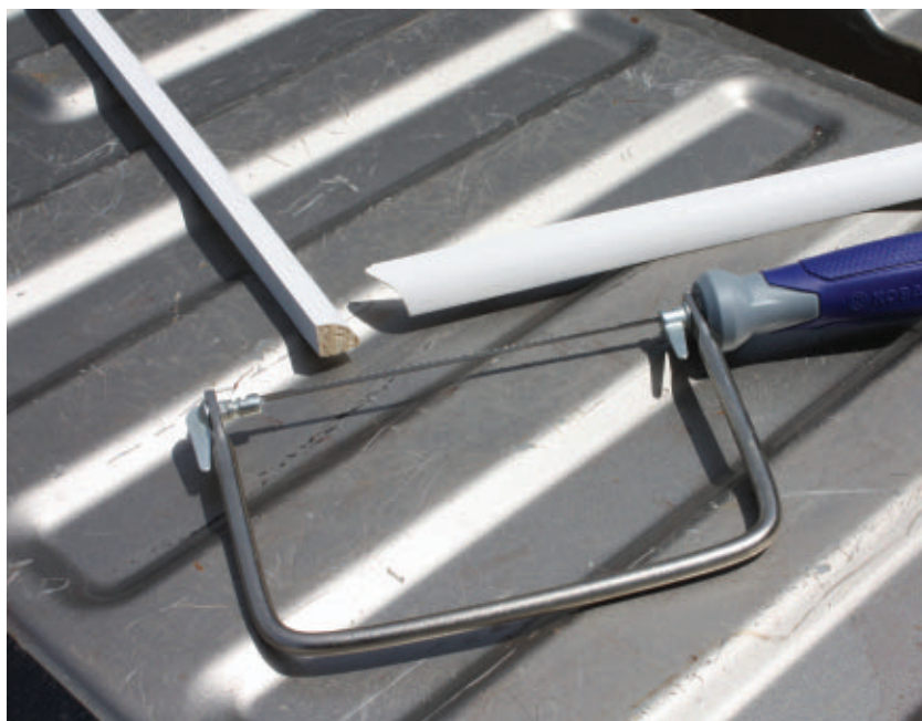
Final step is to install new shoe molding to cover the edges of the floor. I always cut cope joints in shoe molding to ensure a tight fit at the corners.
