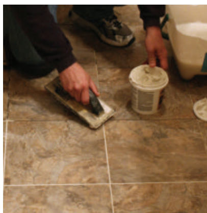
Apply the grout with a rubber float.
