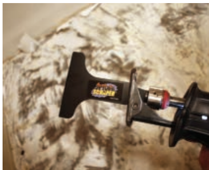
A Spyder scraper attachment for a reciprocating saw speeds up the job dramatically.
