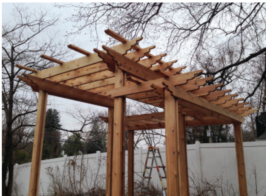
Here's the pergola with all its pieces from the ground up. The combination of posts, girders, rafters and purlins can be modified for almost limitless design choices.
