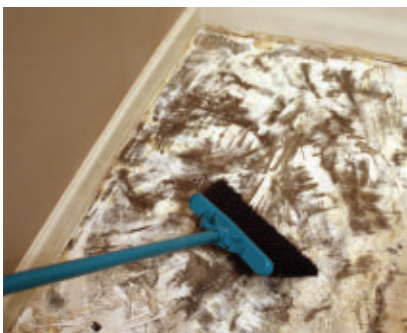
Sweep the floor until it's free of debris and absolutely smooth.
