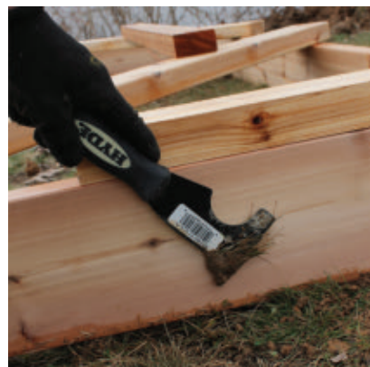
Before moving the template to dig the holes, I gouged its outline in the grass with my multi-tool to help me locate it when it was time to put it back.
