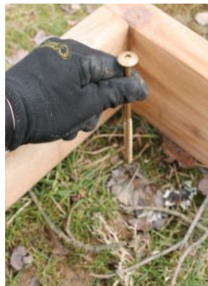
Use screws stuck through a piece of tape to mark the centers of the post holes.
