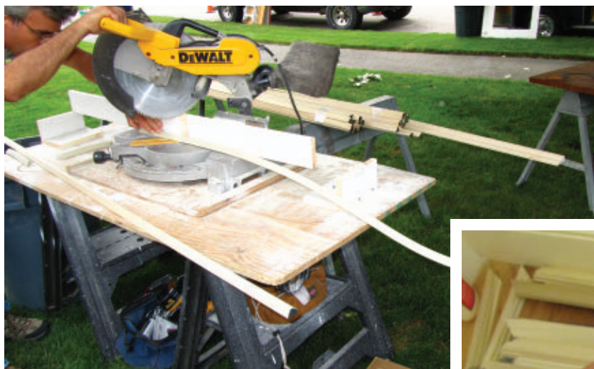
The flexible molding cuts easily on a miter saw.
