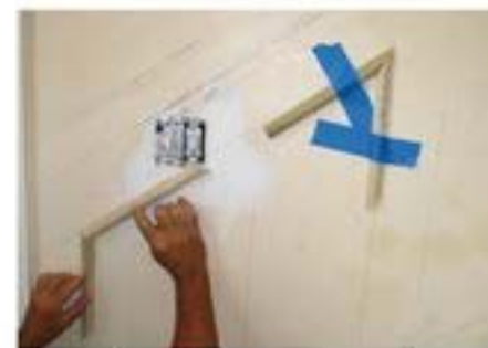
To make this cut you need an acute angle jig (see sidebar).
