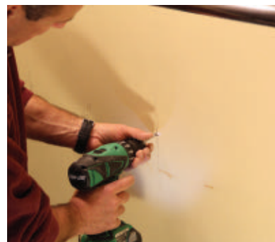
Insulation support rods chucked into a drill are long enough to penetrate the full thickness of the wall and can be seen from both sides. We used the rods to pinpoint the four corners of the tunnel.
