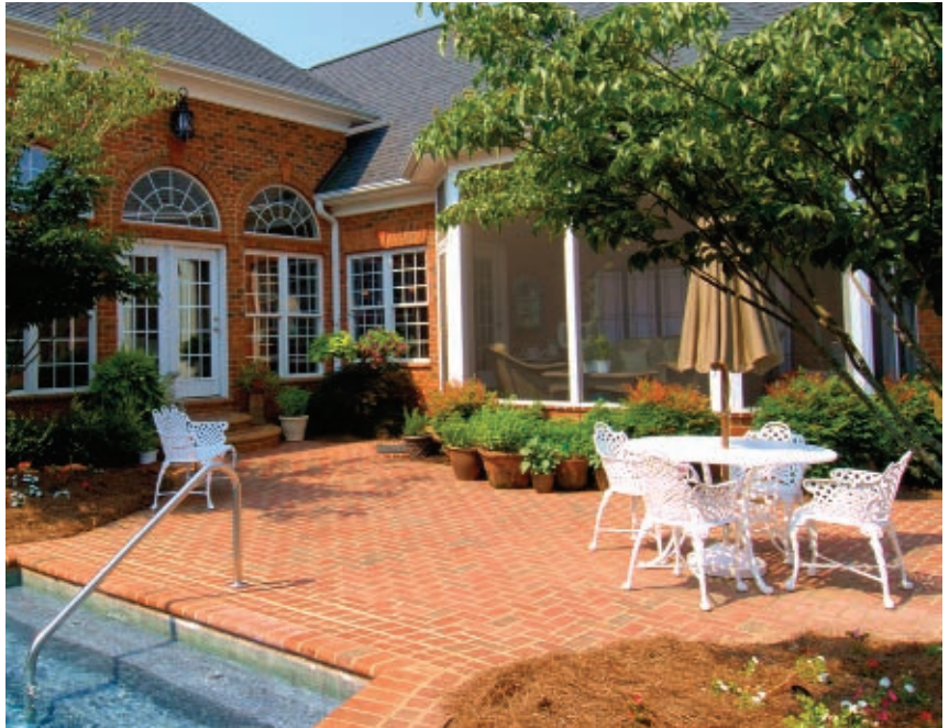
Unlike face bricks, clay pavers are designed for ground usage and engineered to withstand vehicle traffic. (Photo courtesy Pine Hall Brick Co.)
