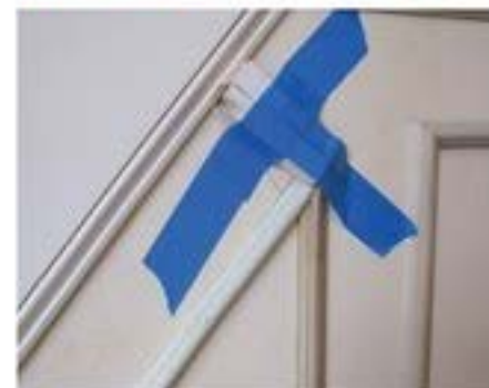
Painter's tape and a wood wedge help hold hard-to-clamp miter joints tight until the glue dries. This is also a perfect place for a spring clamp.
