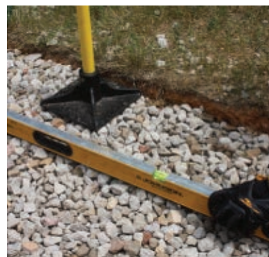
Tamp down and level the gravel bed.
