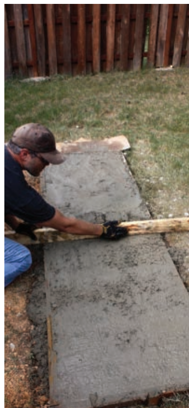
Screed the concrete even with the form.
