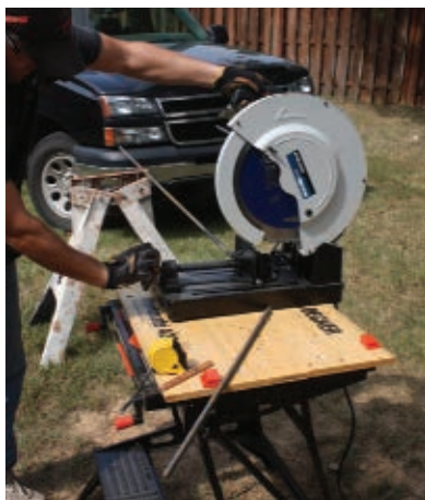
I used a cutoff saw to trim the rebar to size for the reinforcement grid.
