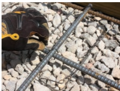
Secure the rebar grid with wire ties.
