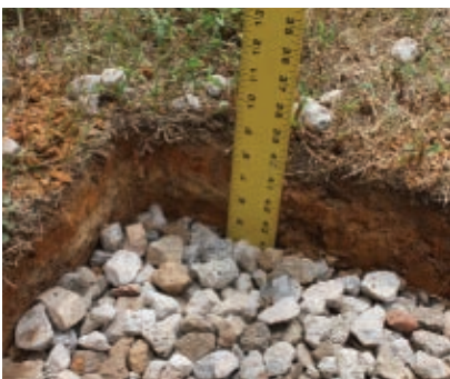
Dig deep enough to account for the gravel base (4" after compaction) and concrete pour (4").
