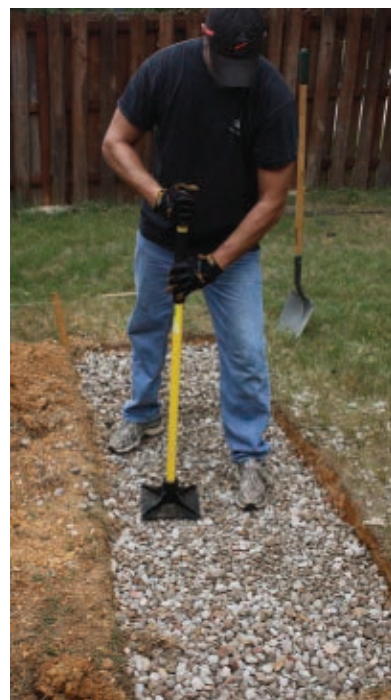
Add a gravel base for the slab.
