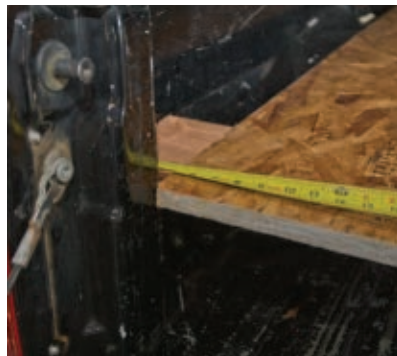
We measured the widest gap and cut a block of wood to match the gap.
