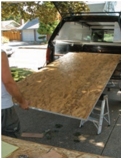
We slid a sheet of 3/4" tongue-and-groove decking into position on top of the cross supports.
