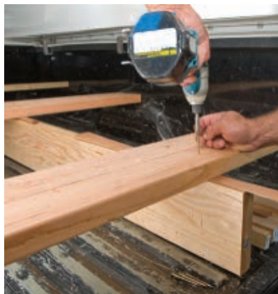
A 2x8 on edge was almost the right height to make a center partition/support running the length of the bed. We used cedar shims to fill the void before fastening the parts with 3" drywall screws.
