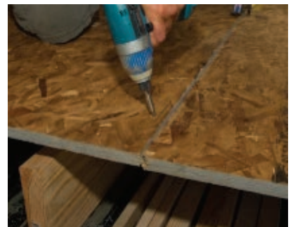
Drywall screws secure the shelf to the cross members.
