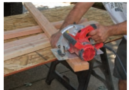
A simple square cut on a 2x4 is all that's needed to make the cross members for the horizontal deck.
