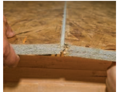
With both pieces in place against the bed walls, we tipped them up at the seam so the tongue and groove could lock together.
