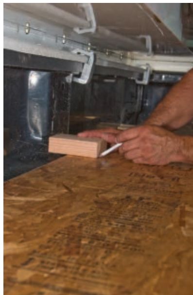
We then used the block as a gauge to scribe the shelf to fit the bed walls.
