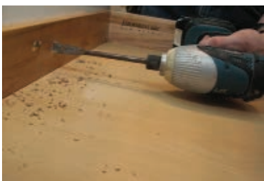
If you're careful you can set hardware screws with a power driver.
