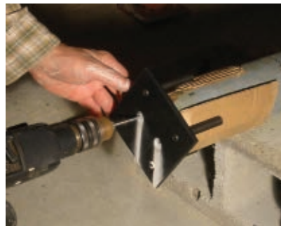
The adjustment plate mounts to the bottom of the column.
