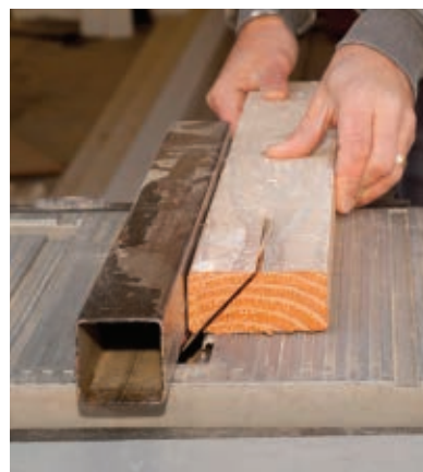
Make the backer blocks by ripping 45-degree triangular shaped strips out of 2x4.
