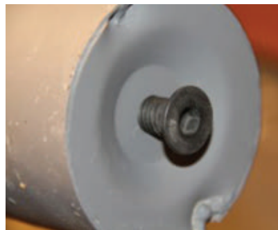
With the screws in place, the cap plate is then removed and mounted to the fastening unit on the Lally Lock column.
