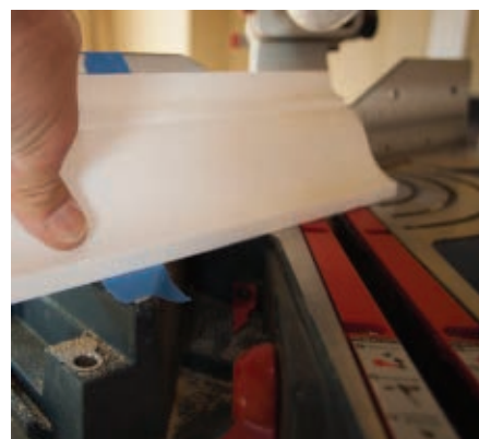
Since the crown goes on the saw upside-down, put the ceiling mark on the table and the wall mark on the fence. Begin a cope cut by making a 45-degree miter back toward the length of the board.
