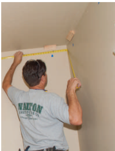
Measure the wall from corner to corner to determine crown length.
