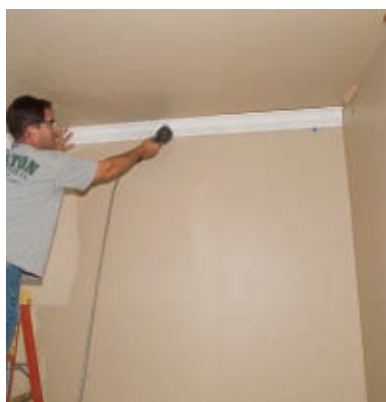
Cut the first strip square on both ends and nail into the backer blocks.
