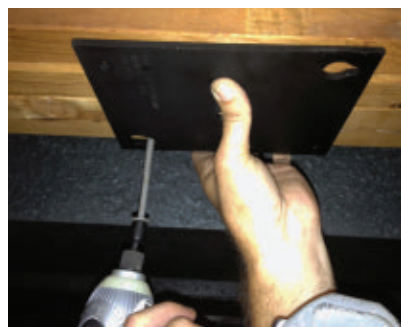
The cap plate is loosely screwed to the beam of the house.
