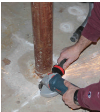
The column must be cut out flush with the foundation floor.
