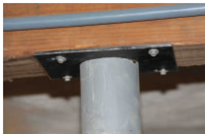
The top plate screws flush and securely to the beam.
