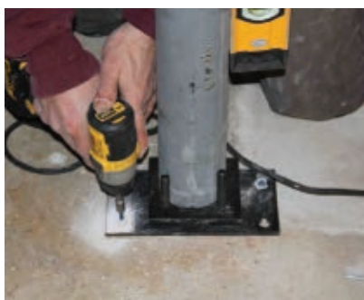
The bearing plate is fastened to the floor with concrete screws.
