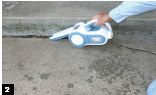
2 Sweep and/or vacuum away all dust and debris.
