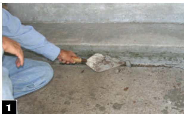
1 The first step is to chip down to solid material and clean away all loose materials and debris.
