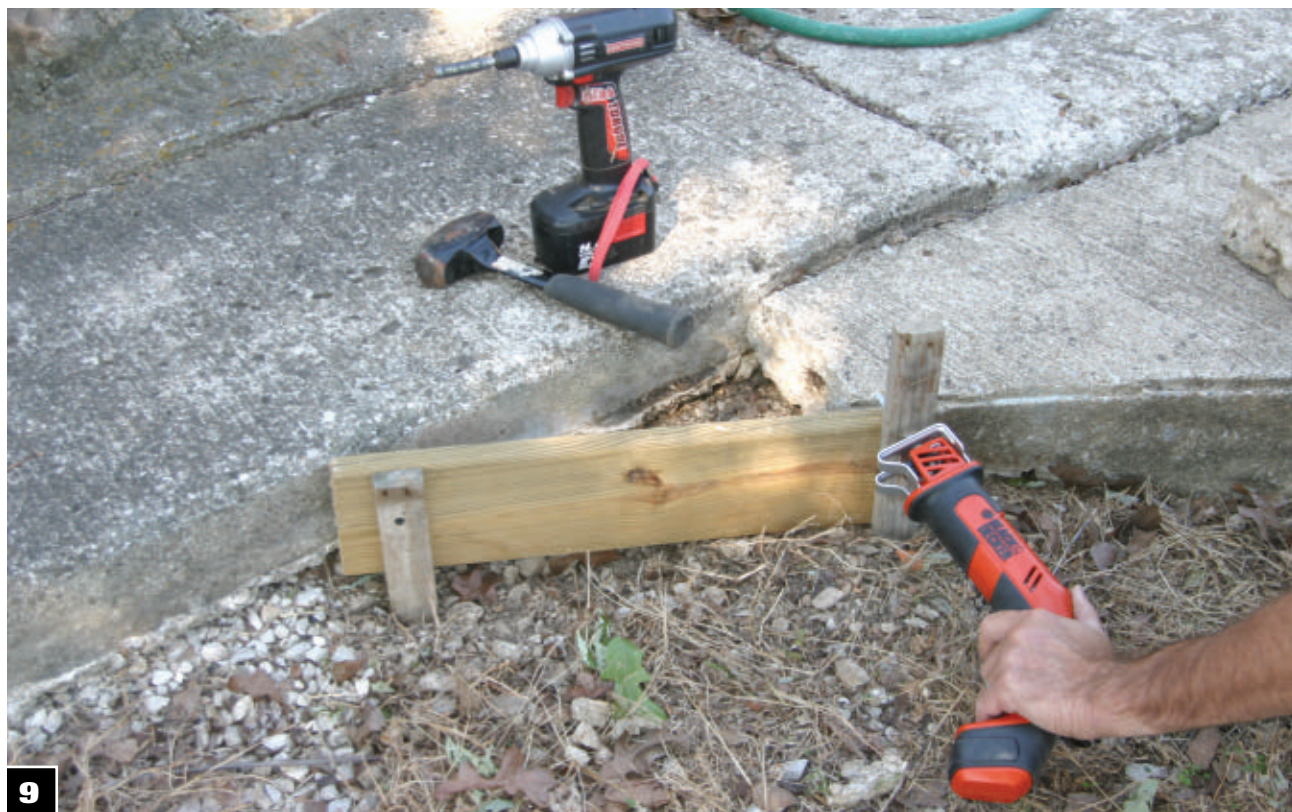
First step is to remove the broken pieces and clean away the debris, then reform to hold the concrete in place. Stakes must be cut flush with the form edge.
