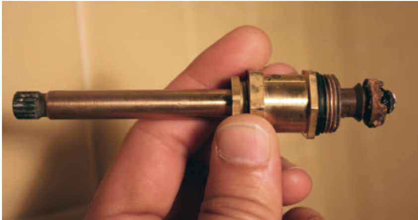
Shown here is the valve stem completely removed.
