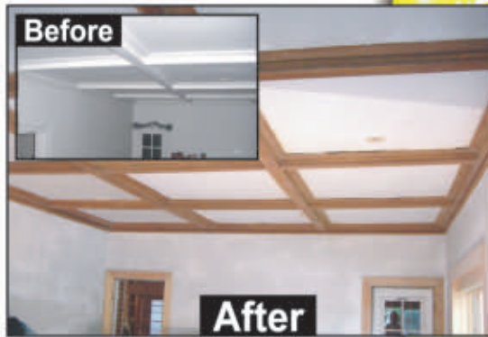
Works on Horizontal and Vertical Surfaces
