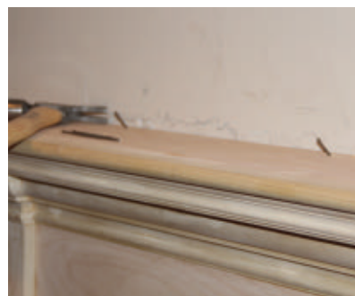
The top was fastened with finish nails toe-nailed into the old nailer.
