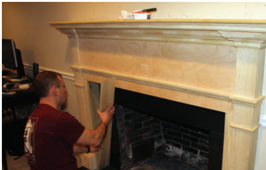
I installed thin trim pieces where the mantel meets the firebox.
