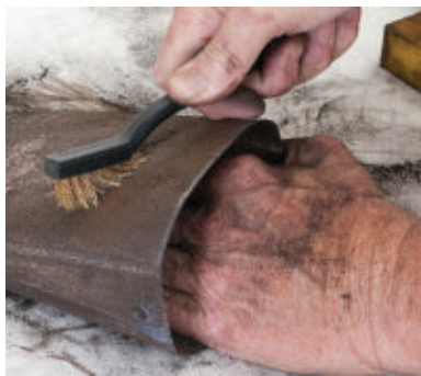
A brass brush can get into the surface pits for a cleaner overall look before painting.
