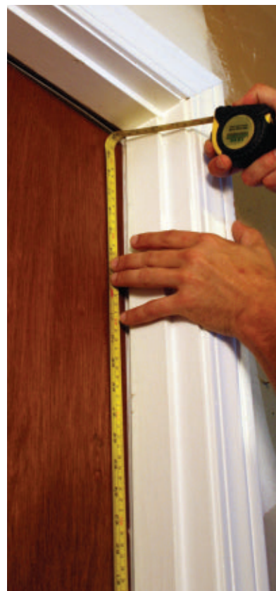
Measure from the door sill to the upper jamb.
