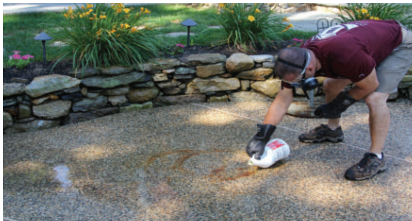
For stubborn stains, reapply the acid to the stain only and repeat the cleaning process.
