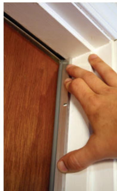
Position the strip against the closed door.
