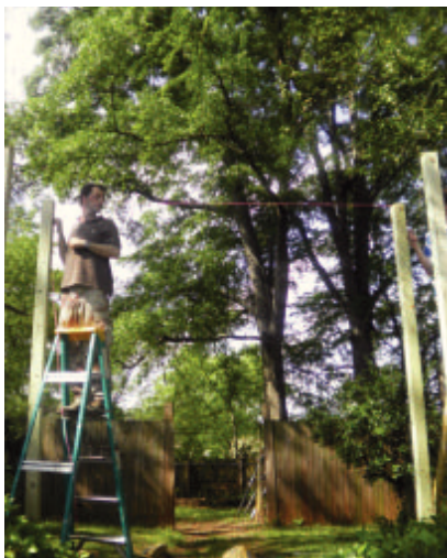
We used a line level on a string to mark the placement of the 2x6 band that surrounds the top of the posts.
