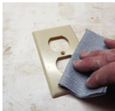
Sand the switch plates with 220-grit sandpaper.
