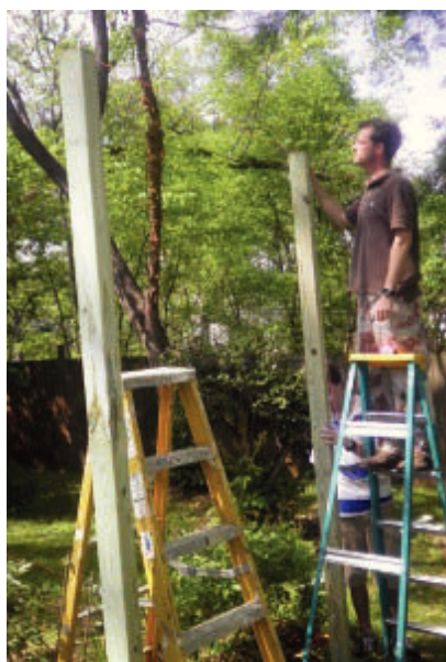
A tightly pulled string helps to keep the posts in line.
