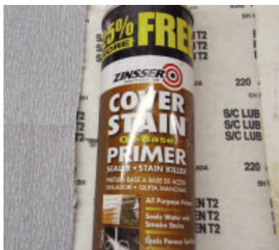
Coat with an oil-based primer.
