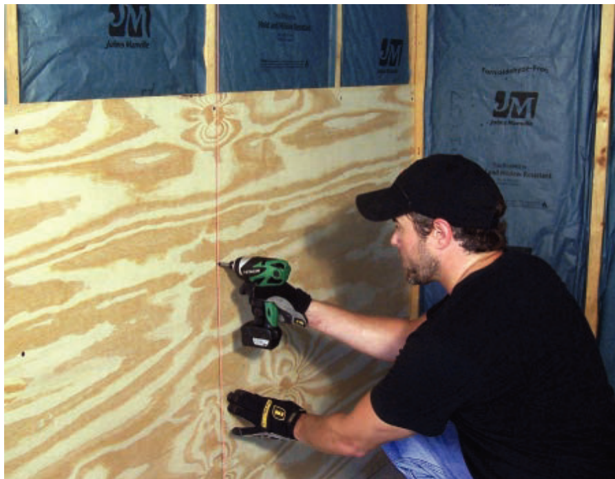
A slat-wall system requires the installation of 1/4" plywood over the wall studs to avoid deflection in the panels.
