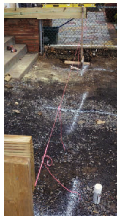
Layout for our mid-span beam was typical. We cut the joists to length, ran a string between and plumbed down for the post locations. On the ground, we marked each hole with a big X to keep on track.
