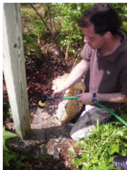
Once you're sure of placement, anchor the posts with quick-drying concrete.
