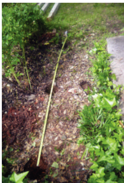
The arbor's post holes were spaced 3' on center.
