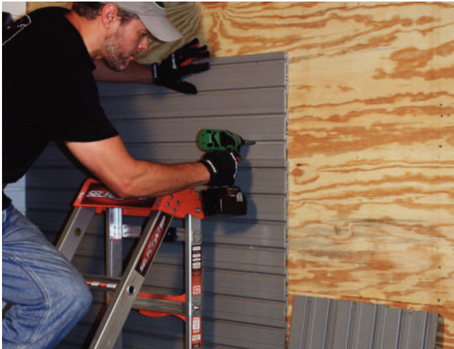
The panels have interlocking edges and install with decking screws driven into the wall studs.
