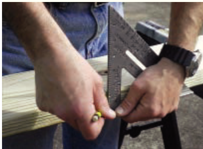
Use a Speed Square to mark bolt locations where the 2x6 boards intersect the posts.
