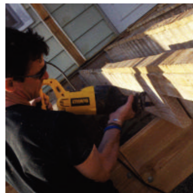
A circ saw along the joists eliminated most of the decking. Using my recip to up-cut the joists halved them quickly and controllably.
