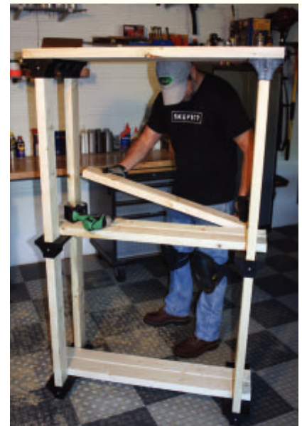
The shelves simply slide over the 2x4 legs. Fasten the shelf brackets in place and then complete the lower and middle shelves by cutting 2x4's to fit between the legs.
