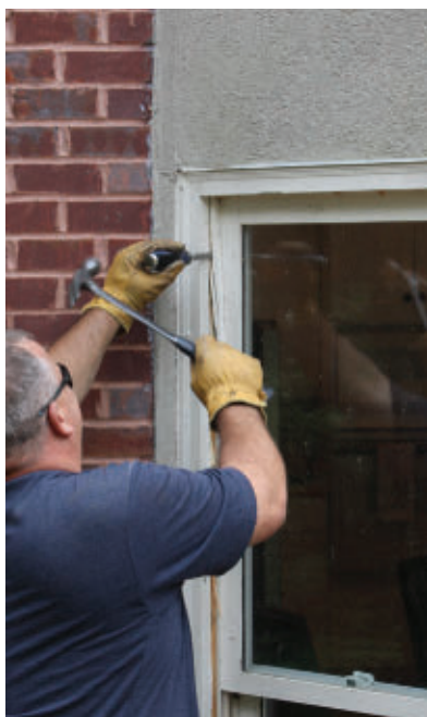
To remove the windows, remove the stop molding along the edges.
