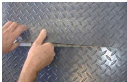
Overlap adjoining edges by 6" or more. Taping the edges and seams is optional.
