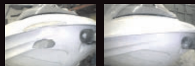
Hull Damage Repair with S-L ASW-01 Anti-Stick White
