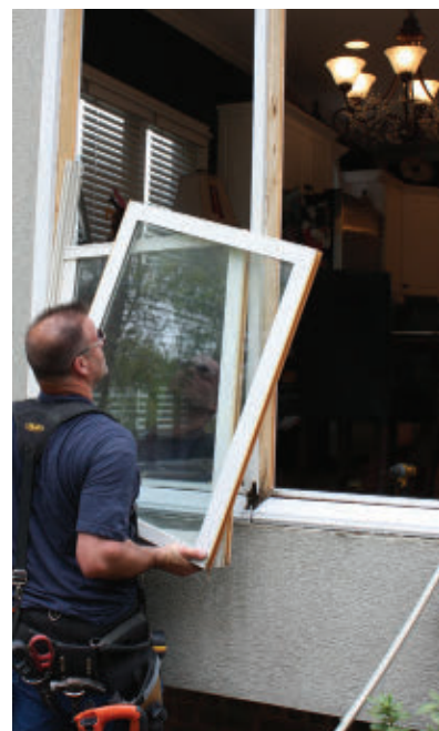
Once the stops are removed the windows can be carefully pulled out of position.
