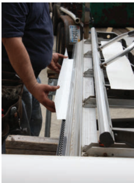
The aluminum trim wrap is fabricated on site to match the size and shape of the wooden window trim.
