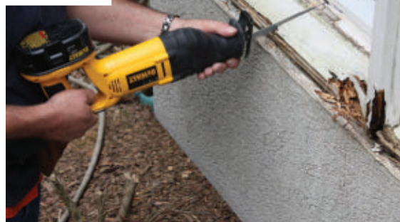
On some windows water intrusion had resulted in sills that were completely ruined by rot.
