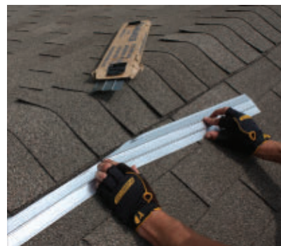
Algae stains on a roof can be removed with the proper cleaning agent and prevented from returning with the installation of zinc strips at the roof ridge.
