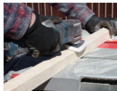
Sand the wood to prep for stain.
