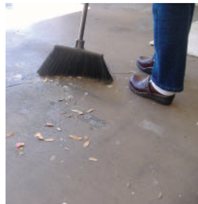
Thoroughly clean the floor prior to installation.
