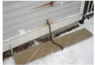
We ran the chain around a large staging plank outside the wall.
