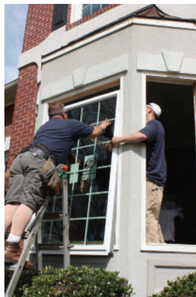
Large units require some assistance when installing. A worker on the inside lifts the window with a suction cup.
