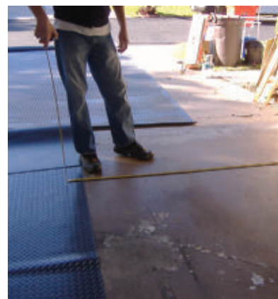
Measure carefully when cutting the floor cover to fit around obstructions.
