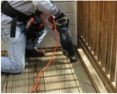
To begin demolition of the decking, I cross-cut the first board with a recip saw.
