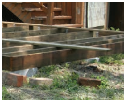
First step is to frame the deck, which is supported on pre-cast concrete pier blocks.
