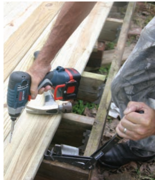
5/4 pressure-treated deck boards are fastened in place on the framing. A Vaughan Bo-Jack makes it easy to take the warp out of boards.
