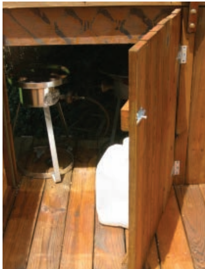
Lower deck boards extend under the deck to provide off-the-ground storage.
