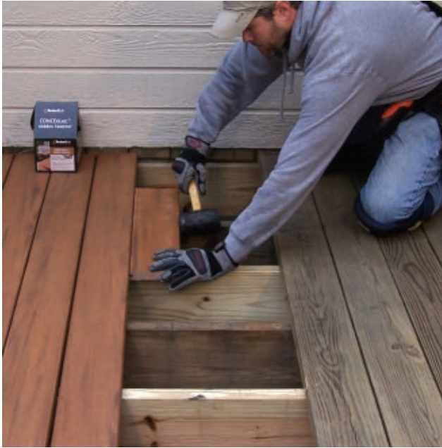
It may help to use a hammer and a scrap of decking to tap the boards together when closing the joints.
