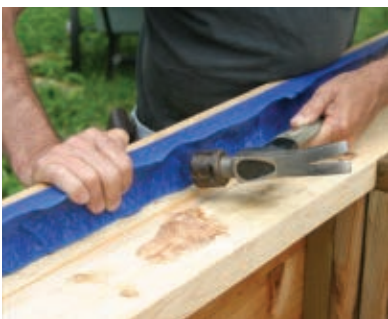
Matcrete 2" splitface Granite Countertop Edge Form is fastened in place with finish nails from the inside.
