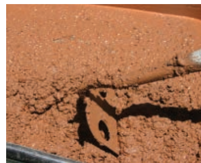
A concrete hoe is used to thoroughly mix the water and concrete.
