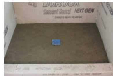
To create a shower floor from scratch, I use what is commonly called "dry pack mortar" or "deck mud", which contains three ingredients; Portland cement, sand and water. The mortar bed is pitched toward the drain.
