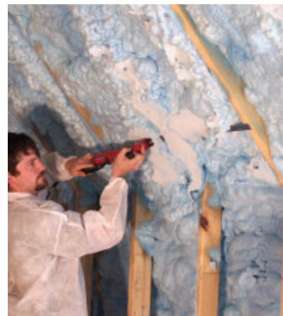
An installer uses a long reciprocating blade to cut the expanded SPF flush with the wall studs.
