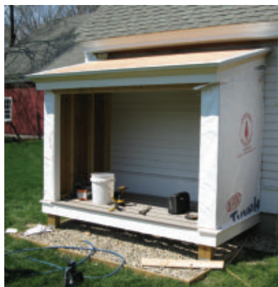
The sheathing was wrapped in building paper.
