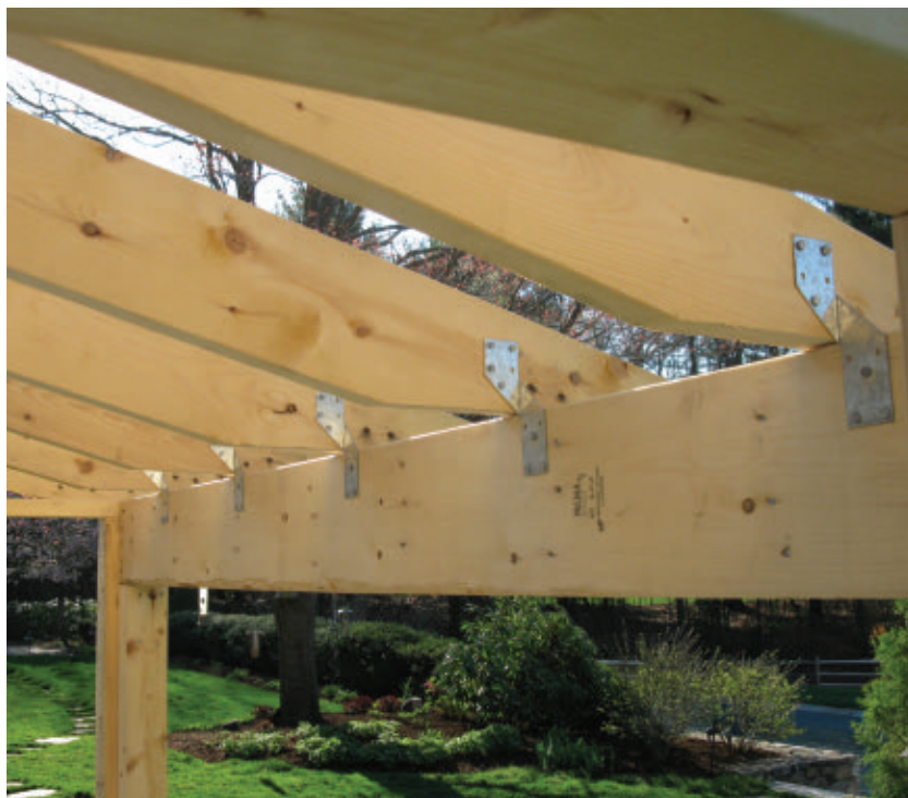
The 2x6 rafters were installed and additionally supported with rafter clips or "hurricane ties".
