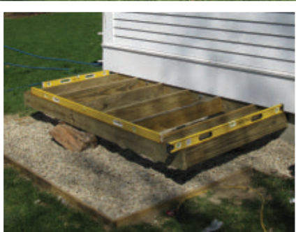
A gravel-covered base lined the foundation.
