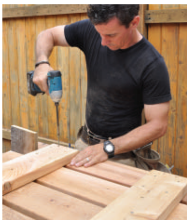
Fasten 2x6 struts to the bottom of the lid with 2-1/2" screws.
