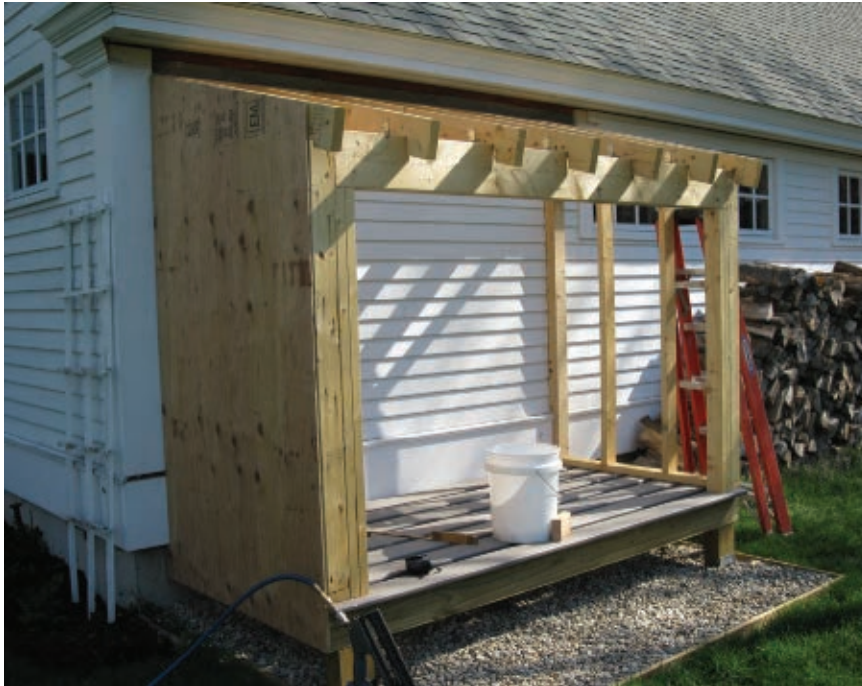
The walls as well as the roof received 1/2-in. CDX plywood sheathing.
