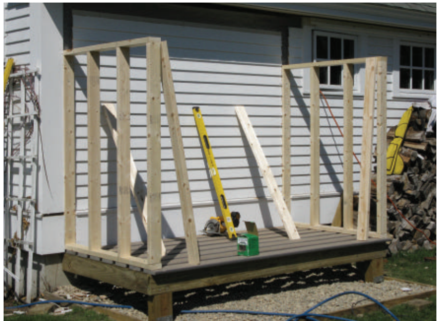
We used regular 2x4 Douglas fir studs 16-in. on center for the wall framing, and built the walls tall enough to accommodate a 3- to 4-pitch roof.
