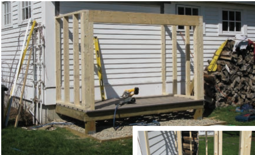
A 2x10 double header carries the roof load over the wood shed opening.
