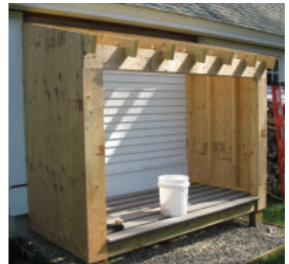
We secured wall and roof sheathing with 8-penny ring-shank nails every 10" in the field and every 6" at seams and edges.
