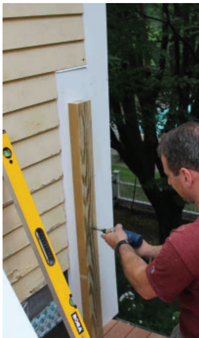
A 2x4 was used as the framing for the half post sleeve.
