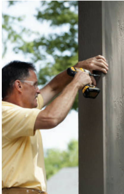
Attach the column wrap with non-corrosive fasteners.
