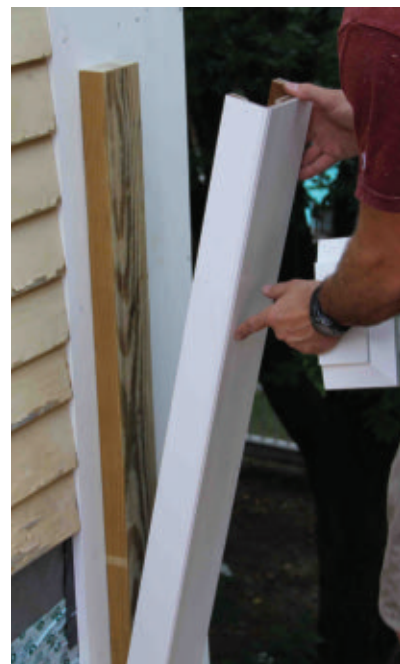
The halved sleeve slips right over the 2x4.
