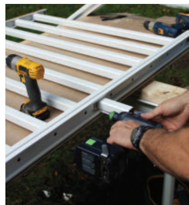
The balusters are easy to fasten through channels in the upper and lower rails.
