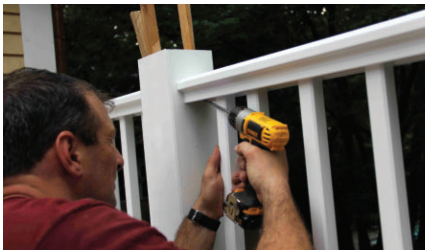
The fasteners are concealed within the rails for a finished look.
