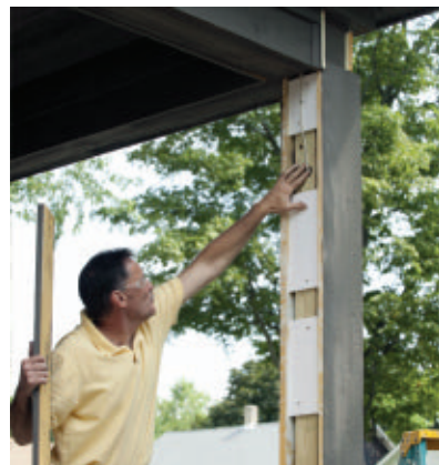
Dry-fit the column-wrap components to make sure no further adjustments are necessary.
