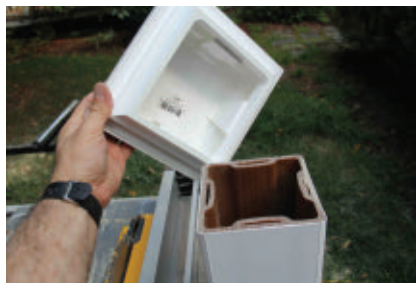
The posts are trimmed with a post cap at top and a post skirt at bottom.
