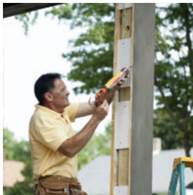
Apply premium construction adhesive to the joint.
