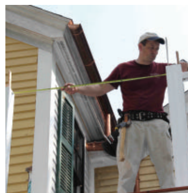
Measure between posts to determine length of your rail sections.
