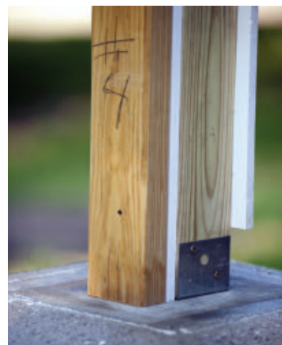
Blocking was added to the post to provide a solid nailing surface.
