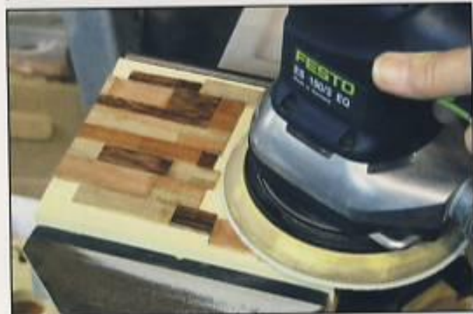
Step 10. Using the orbital sander, sand the overlays to obtain a smooth, even surface.
