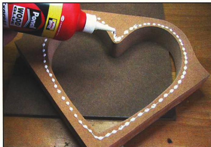
Step 10. Apply wood glue to the bottom surface of the box body.
