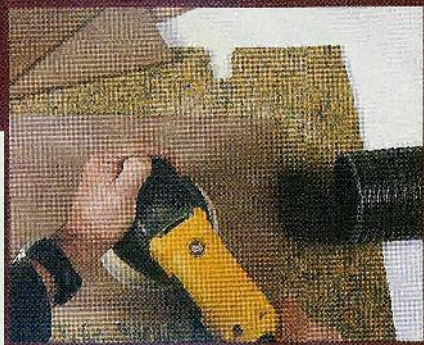
Step 2. We move on to a random orbit sander with 120-grit paper.
