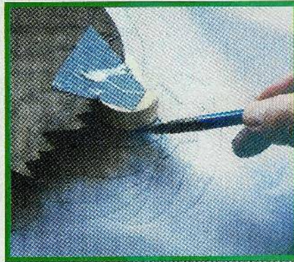
Fig. 2. Use duct tape to hold the pieces together.
