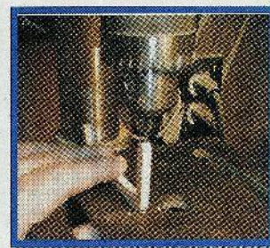
Fig. 11. Drill a hole for the screw eye.
