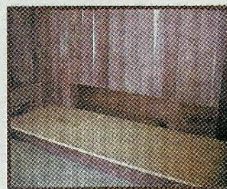
Fig. 9. Secure the bottom shelf to the bottom supports.
