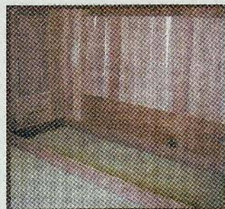
Fig. 7. The bottom supports are attached and ready to receive the shelf.
