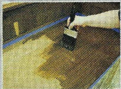
Cindy brushes on seal-coat of EnviroTex Lite to seal the wood prior to final pour.
