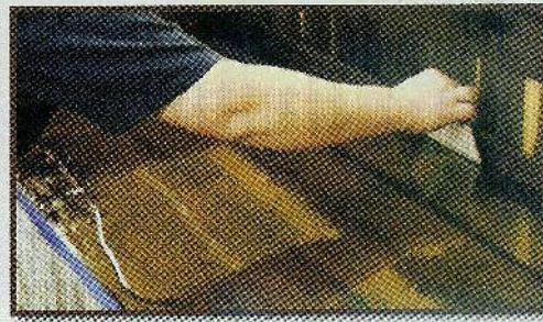
Fig. 24. Push the Envirotex to the edges of the bar top with a spatula.
