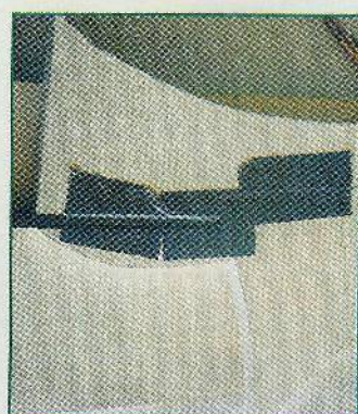
Fig. 4. Duct tape can be used to temporarily join the pieces as they are cut.
