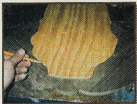
Step 10. Use the cut plywood piece as a template to fit the shoulder pieces.
