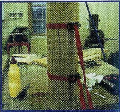
Fig. 3. Clamping up the hexagonal column.
