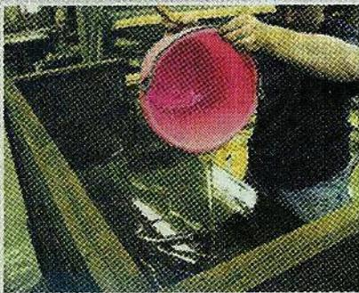
Cindy does the final pour of EnviroTex Lite® on the bar's work surface.
